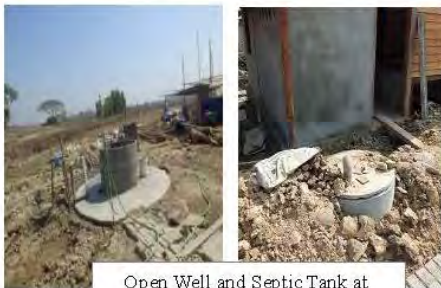
Open Well and Septic Tank at Relocation site
