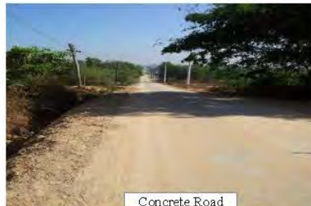
Concrete Road Paved
