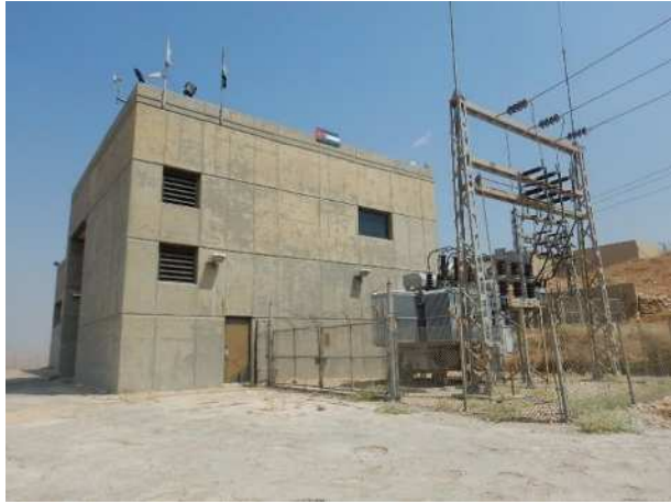
Raw water pumping station
