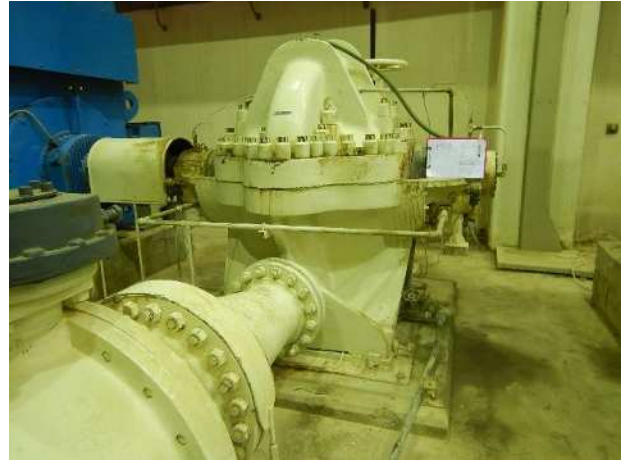
Single-stage centrifugal pump
