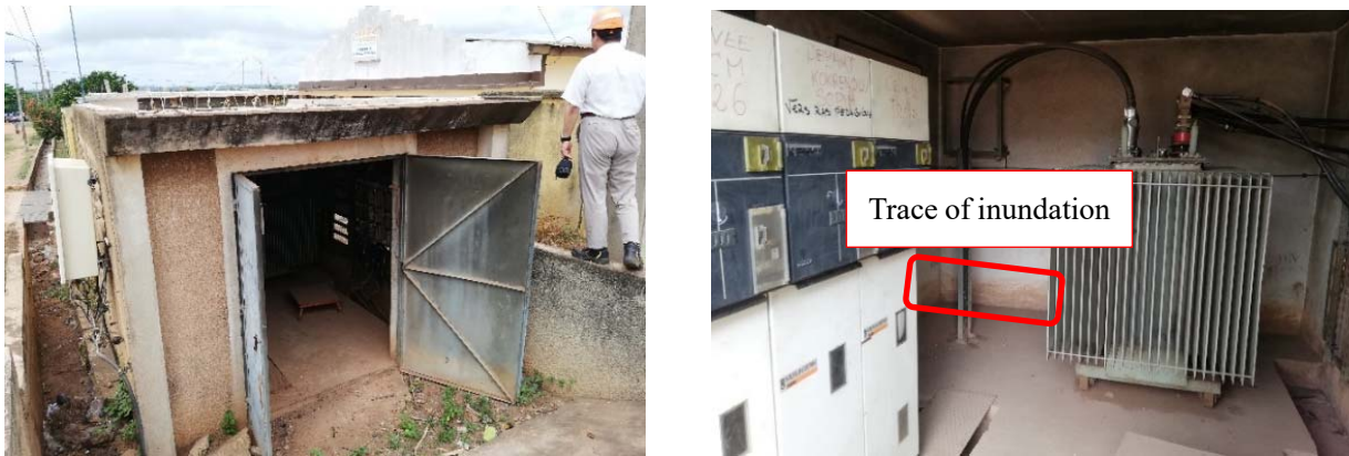
Fig. 6.4-11 Existing post P148
