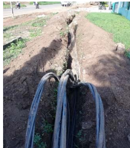
Fig. 4.3-2 Underground system (under construction)
