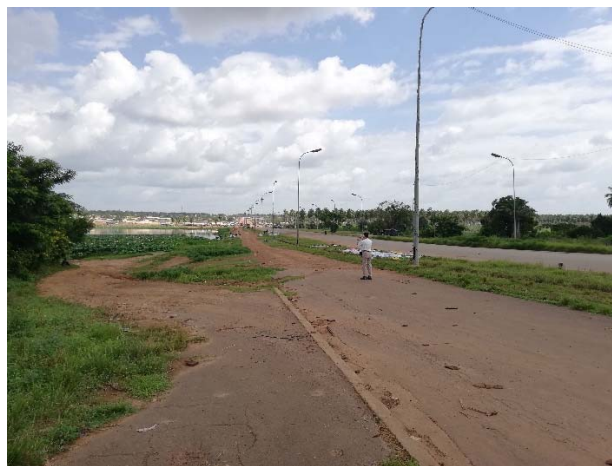
Fig. 4.3-10 The road at the city center of Yamoussoukro (crossing the pond)
