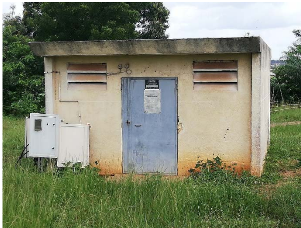
(Building of distribution substation)
