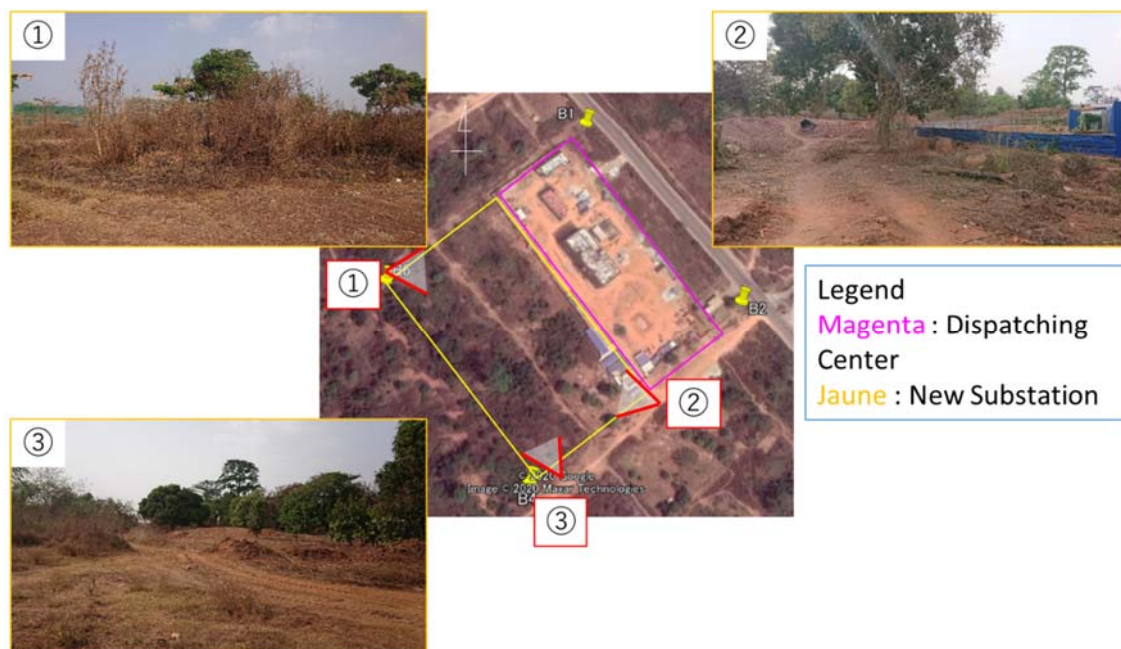
Fig. 4.2-1 The candidate site of Yamoussoukro 2 substation
