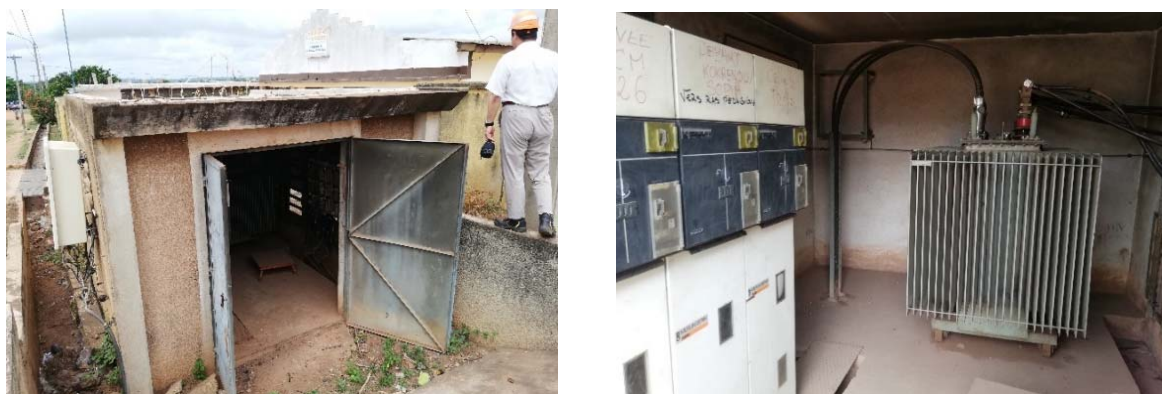
Fig. 4.3-13 Distribution posts at risk of inundation
