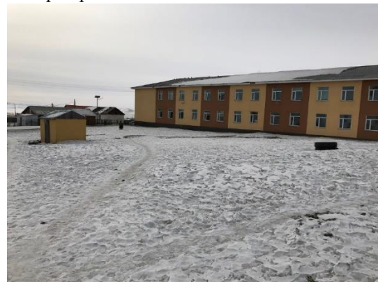
Installation site of geothermal exchanger (next to the school building)
