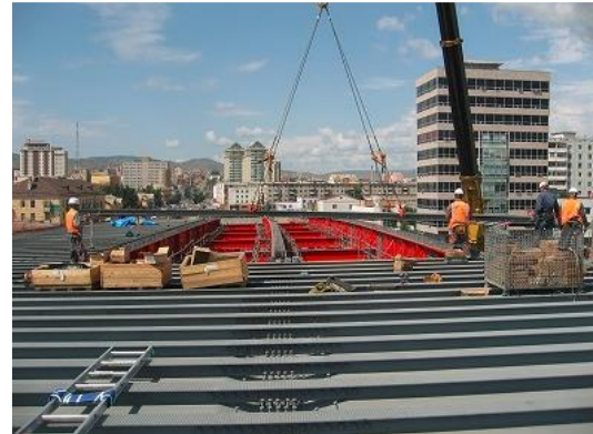
Construction of Composite Deck Slab
