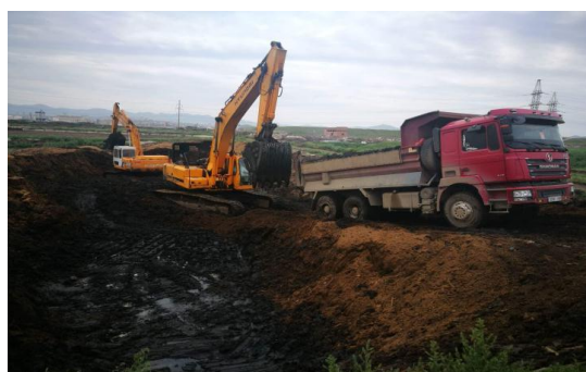
Removal of Accumulated Sewage Sludge
