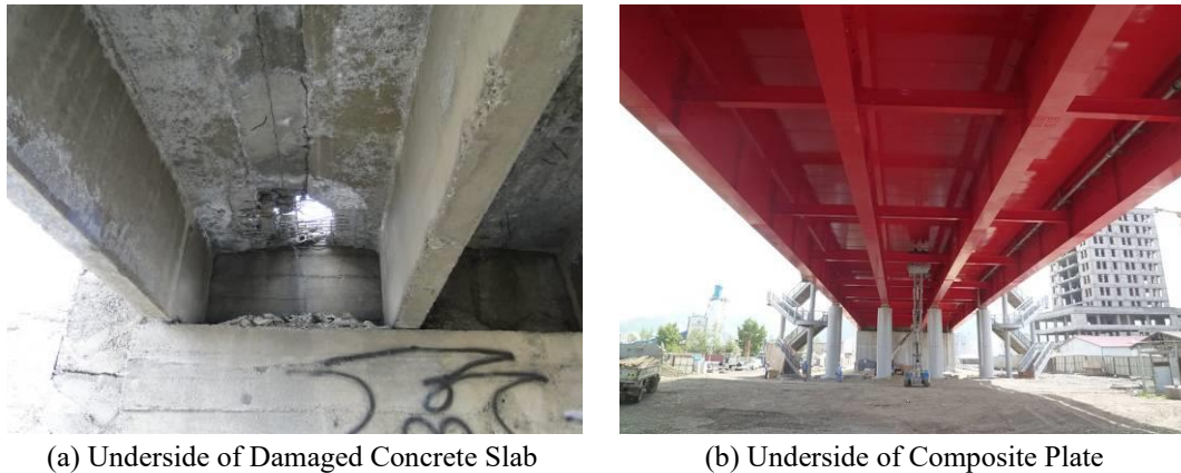
Figure 3.8 Bottom of Slab
