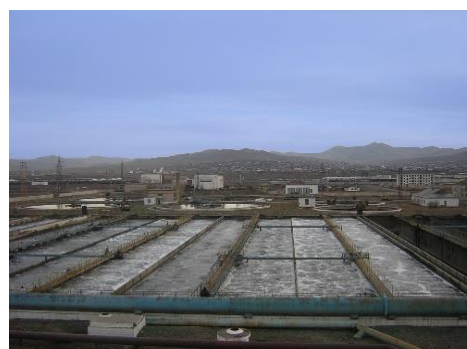
Wastewater Treatment Facility
