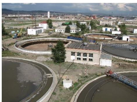
Primary Settling Tanks
