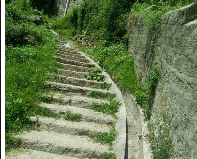
No. 11: Existing cement concrete channel along the village path.
