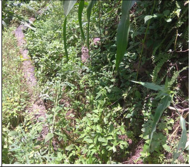
No. 8: Existing cement concrete distribution channels
