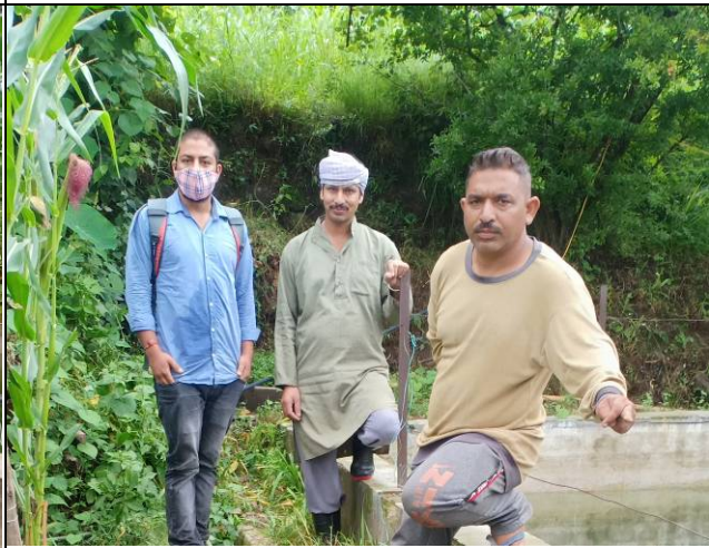
No. 6: Existing cement concrete channel.
