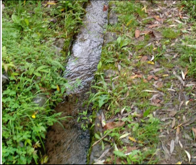
No. 7: Existing cement concrete channel
