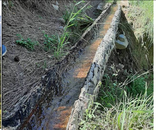
No.8: Existing channel of Chir Pine made by farmers for taking water for irrigation.
