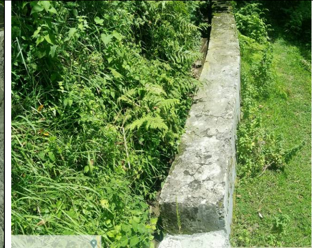
No. 12: Existing water channel.
