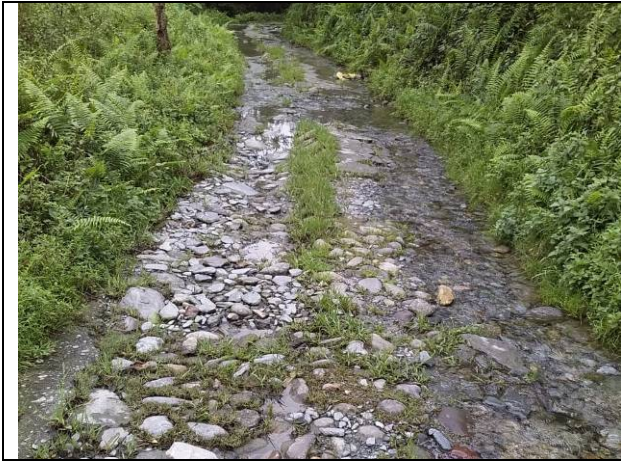
No. 7: Existing Kutcha Farm Access Road approx. length 2 Km.
