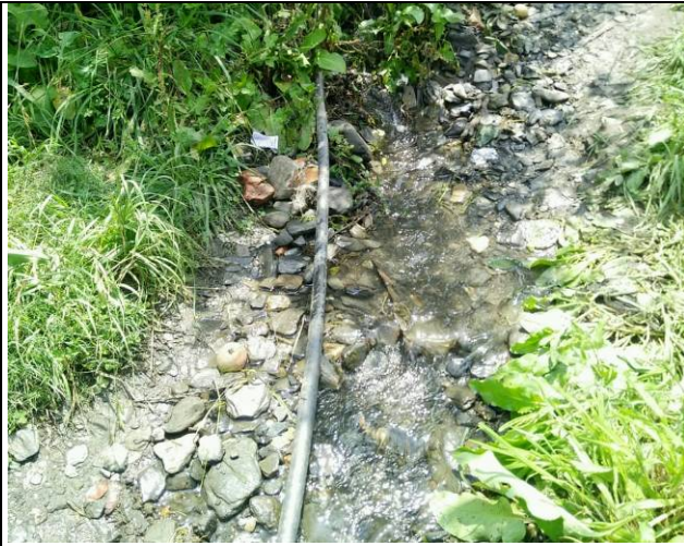
No. 11: Existing Kutch channel used for taking water to the CCA.
