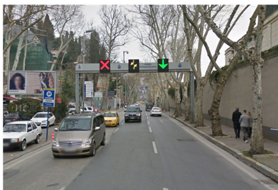
Image of the reversible lane operation and signal installation in Links Rd three-lanes section
