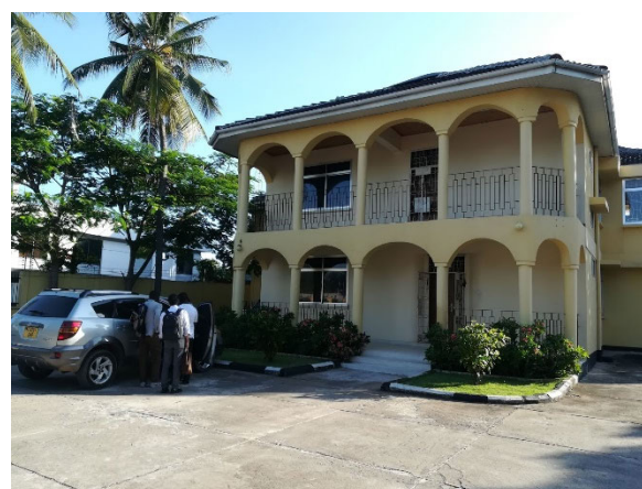
The VTC building. The monitoring room stations are on the ground floor level. No-frill operation.
