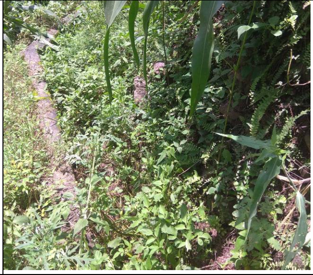
No. 8: Existing cement concrete distribution channels
