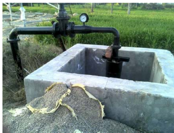
View of the laying Shallow Tube Well in HPCDP
