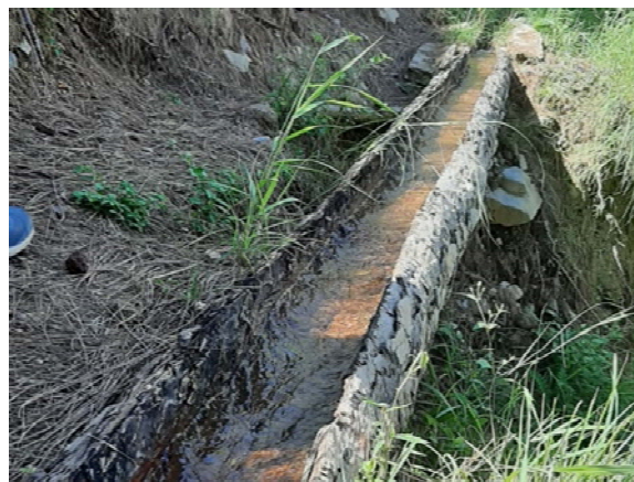
View of the field survey on existing channel of Chir Pine made by farmers for taking water for irrigation at village Ghara, G.P nerwa, District Shimla
