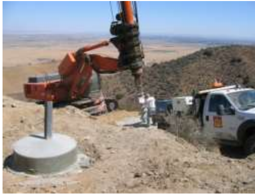
Figure 3.3-1 Illustrative Photo for Construction of Transmission Line Foundation
