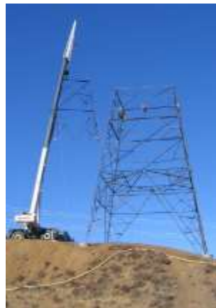
Figure 3.3-2 Illustrative Photo for A Crane Carrying the Top Section of Tower for Installation
