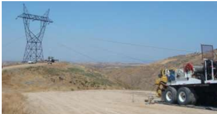
Figure 3.3-3 Illustrative Photo for Pulling phase of a wire-stringing operation
