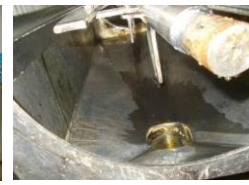
Water residues in processing line
