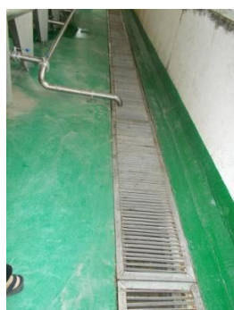
Floor inclined to drains
