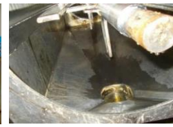
Water residues in processing line
