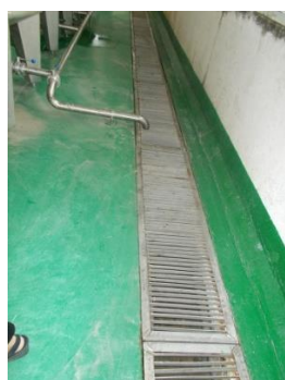
Floor inclined to drains
