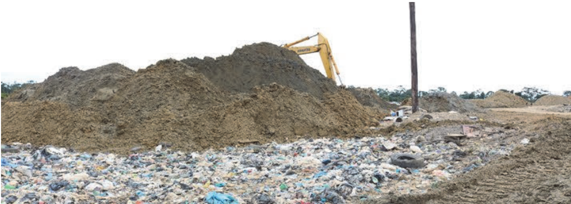
Figure 2-28 Soil cover operation in the Ornamibo final disposal site in the Republic of Suriname (Photograph) 49
