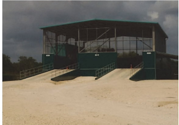
Burrell Boom Transfer station
