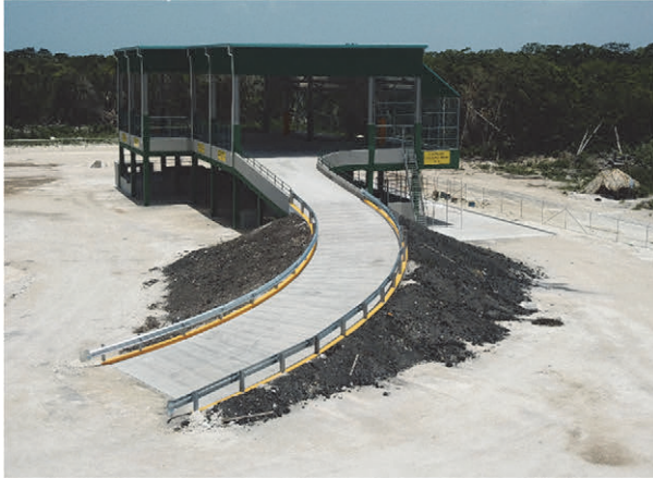
Corozal Transfer station
