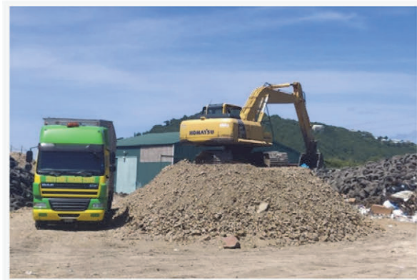
Vieux-Fort final disposal site
