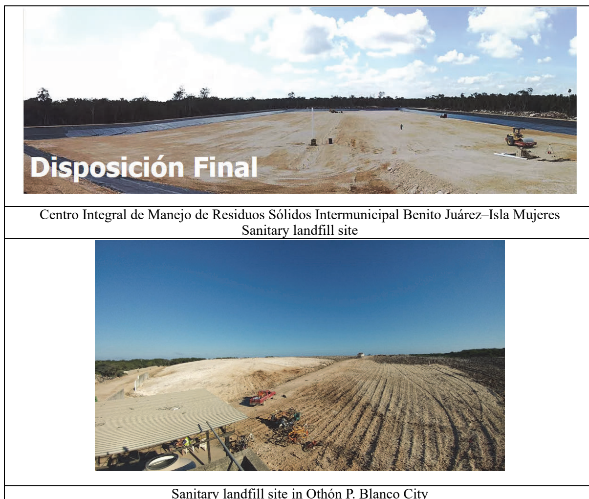
Figure 2-64 Sanitary landfill sites in Quintana Roo (Photographs)
