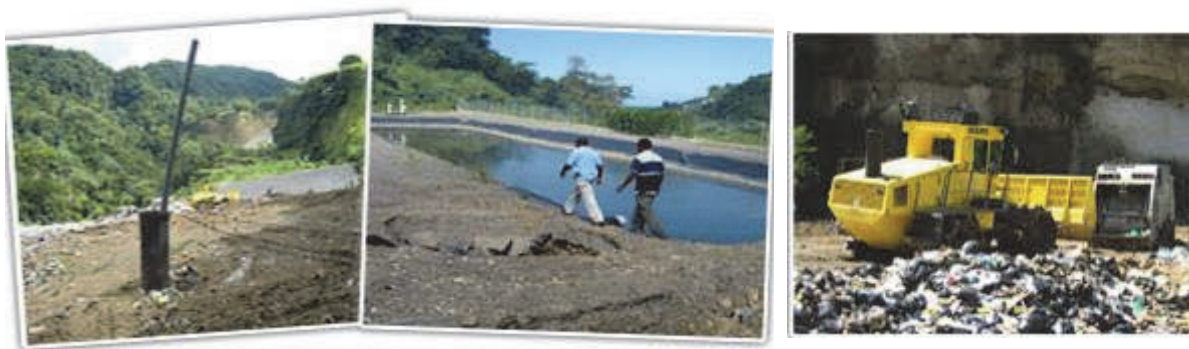
Gas extraction pipe and leachate treatment facility
