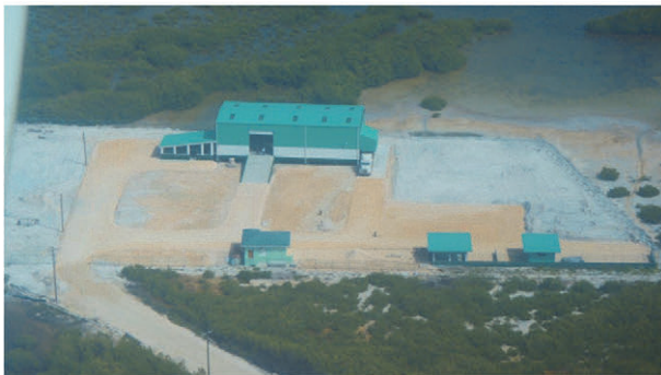
San Pedro transfer station
