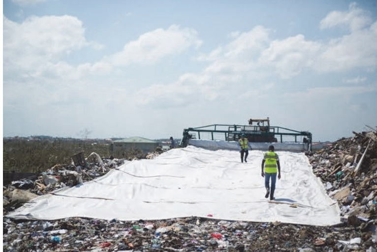
Figure 2-14 State of Haags Bosch final disposal site in the Republic of Guyana (Photograph) 29
