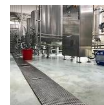
Floor with drainage for washing
