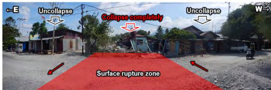
Figure 38 : Collapse of the house on the surface rupture zone at 20181102-10 site
