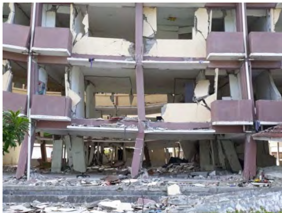
Figure 50 : Out-of-plane wall and column sway mechanism
