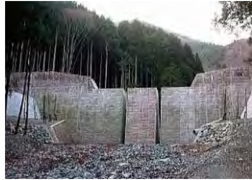
Check SABO Dam (WASHINO SAWA in Japan)
