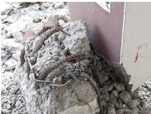
Figure 56 : Non-deformed bars still used
