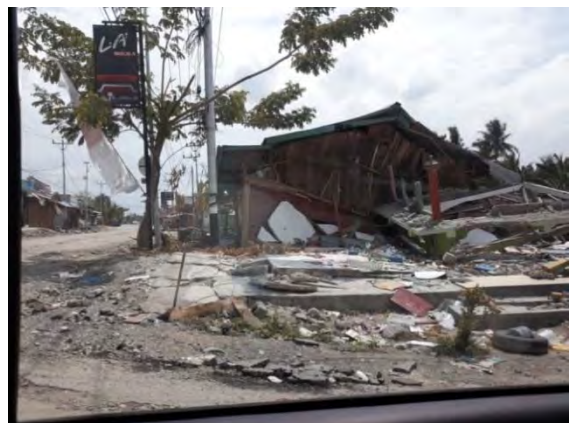
Figure 63 : Total Collapsed of House
