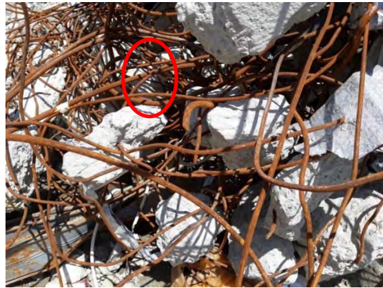
Figure 55 : Non-deformed bars still used in Lere,
