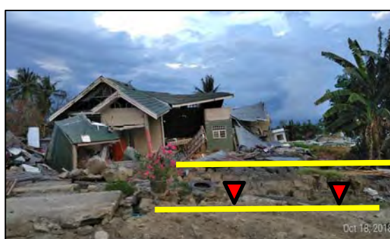
Figure 67 : Collapsed by Land Subsidence
