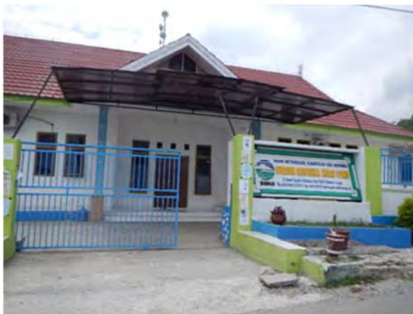
Figure 44 : Palu class 1 geophysical station
