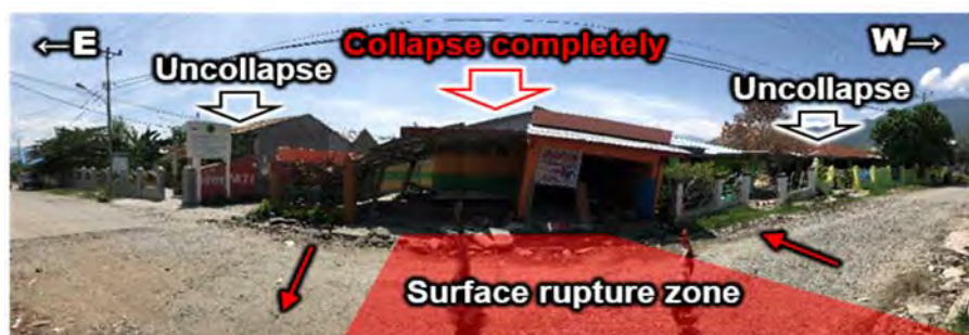
Figure 37 : Collapse of the house on the surface rupture zone at 20181103-3 site
