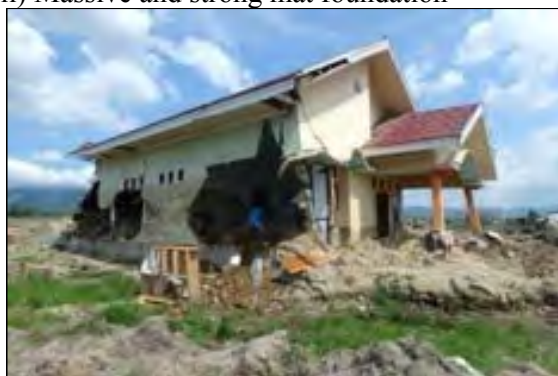
Figure 105 : Unmoved house with massive foundation in Jono Oge liquefaction damage area and image of liquefaction-landslide resistant building
