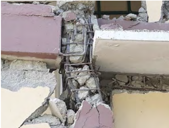
Figure 52 : Joint failure
