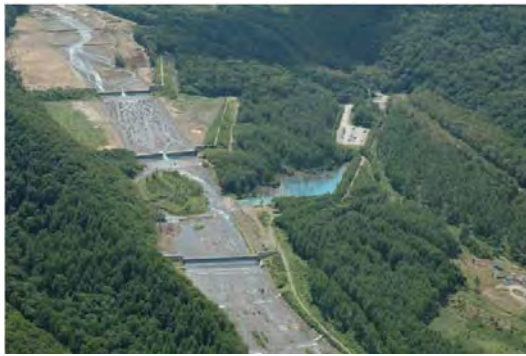
Revetment, Series of Consolidation Dam or Ground Sill Work (BIEI River in Japan)
