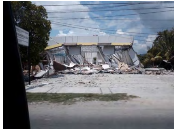
Figure 59 : Collapsed of Store
