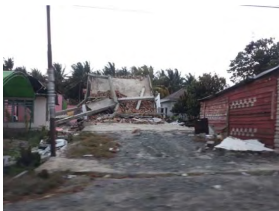
Figure 64 : Total Collapsed of House
