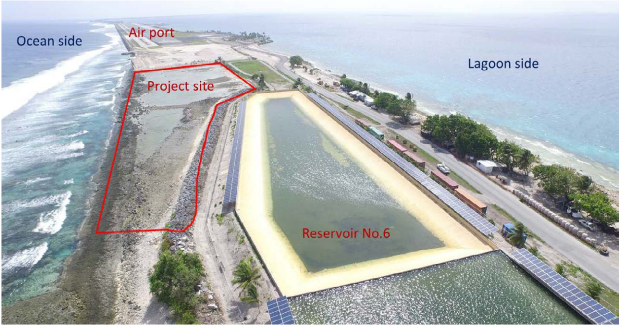
Construction site for the Project
