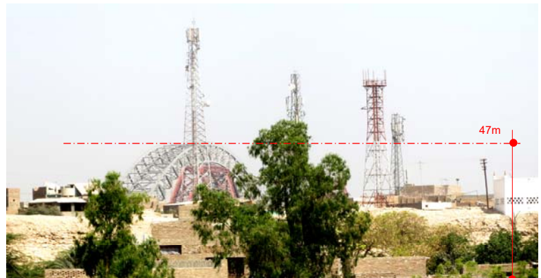
Ground level is 4m higher than the proposed Project Site + Height of Lansdowne Bridge 43m = 47m + 1m Clearance = 48m
