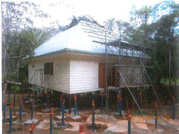
Plate 1. External view of the Visitor Information Centre
