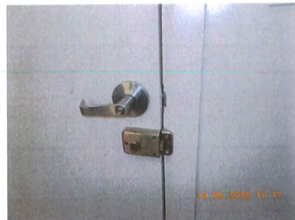
Plate 10. Door furniture to the external doors
