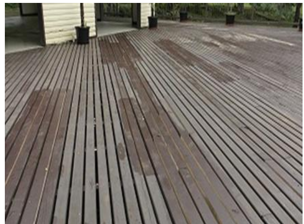
Photo 6: Wood decking at ICC was repaired by park rangers (VNP).
