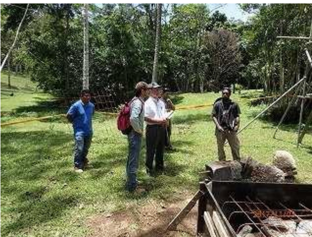
Photo 5: Mr. Sakano and Mr. Imai of JICA inspecting progress at the construction site of new information center (VNP).
