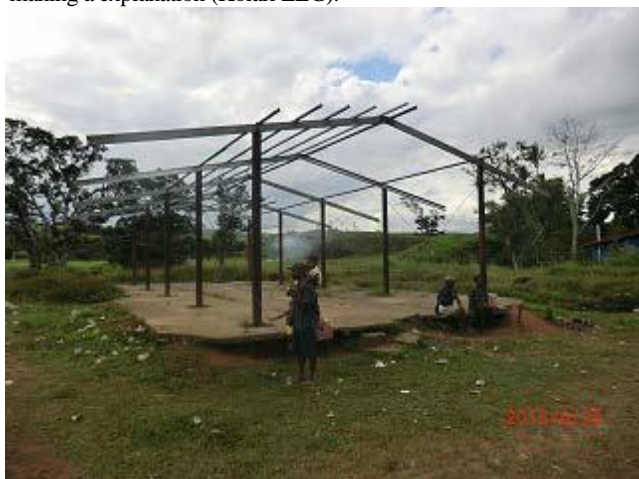
Photo 3: Sogeri Local Market construction site (Koiari LLG).
