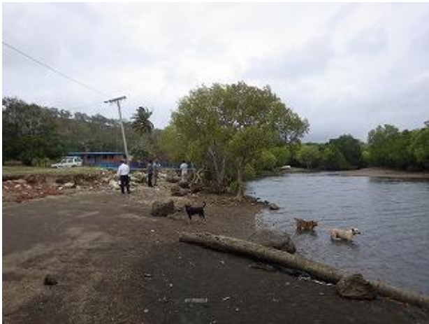
Photo 7: CEPA-JICA project, checking condition of the site at Mirigeda damaged by coastal erosion (Port Moresby).
