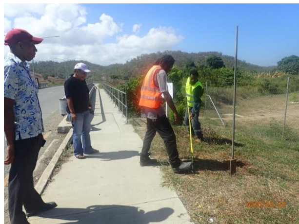
Photo 2: CEPA-JICA project team, checking installation site of the signboard for output 3 (Central Province).
