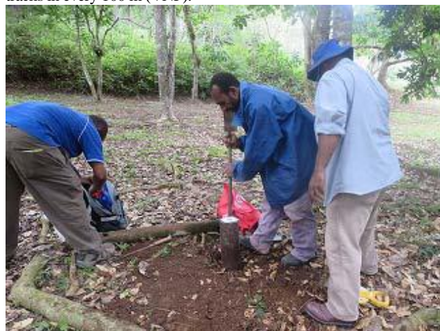
Photo 4: Work for distance pile installation. (VNP).
