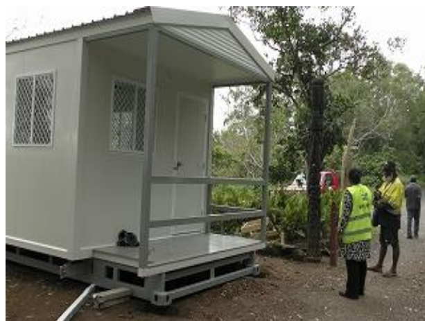
Photo 6: New tall gate house was established at the entrance of Varirata National Park (VNP).
