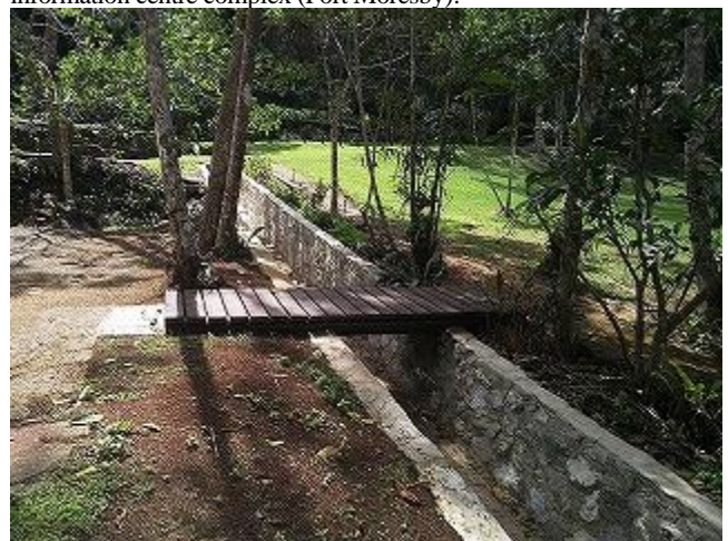
Photo 4: Newly installed trench and wooden foot bridge, ready to be used by visitors (VNP).
