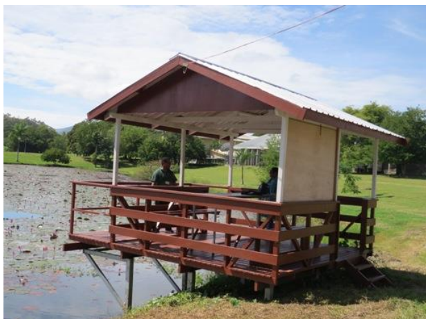
Photo 1: Extension work of the bird watching shelter at Pacific Adventist University was completed (PAU).
