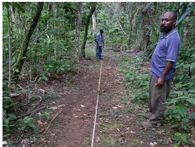
Photo 2: JICA Technical Coordinator, Mr. Ted Mamu, supervising installation of distance piles at VNP. Piles were installed along all tracks in every 100 m (VNP).
