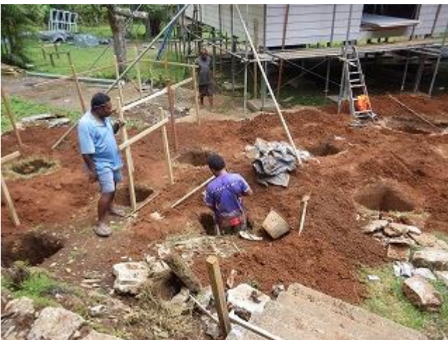
Photo 11: Local contractor digging holes for installing support piles of wood deck (VNP).
