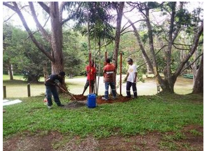
Photo 6: Construction workers installing main signboard at the main picnic area (VNP).
