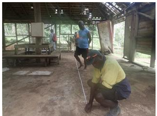
Photo 6: Local construction company has conducted a field survey for proposing renovation of the Information Center. (VNP).
