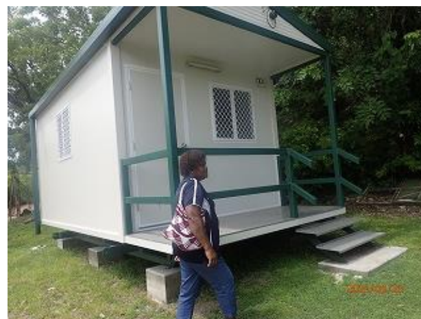
Photo 4: CEPA-JICA Project Team, inspecting marine station office installed by API at Tahira (Tahira).
