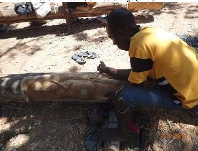
Photo 5: A local craftsman making a totem pole with cultural base-relief for renovation of old Information Center at Varirata National Park (Port Moresby).
