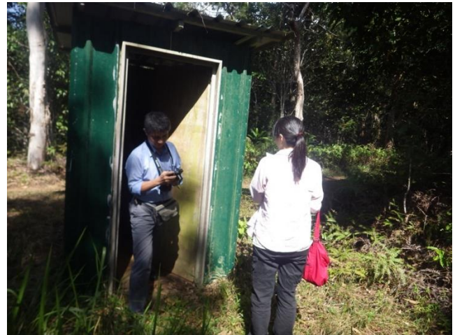
Photo 10: Dr Imae and Ms Ayako inspecting the conditions of the toilets at VNP (VNP).
