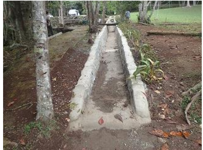
Photo 2: Repairing the drainage in Varirata National Park has successfully been completed (VNP).
