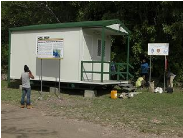
Photo 7: Two signboards for Tahira marine station were installed (Tahira).
