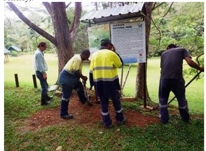
Photo 6: Mr. Imai of JICA, supervising the contractors installing a signboard at the main picnic site of the park (VNP).
