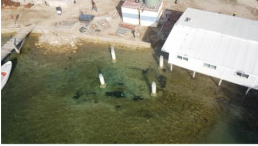
Dive Shop Foundation completed
