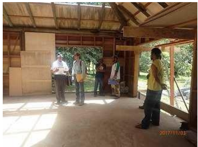
Photo 6: Mr.Sakano and Mr. Imai of JICA inspecting progress of renovation of old information center (VNP).
