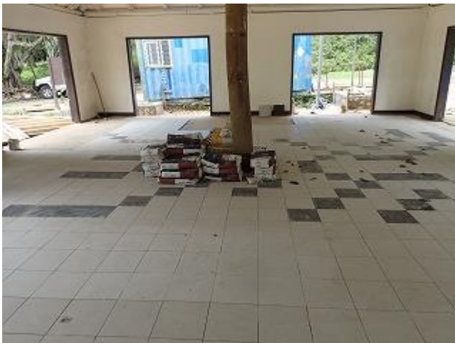
Photo 3: Tile installation progressing for renovation of Old Information Center (VNP).
