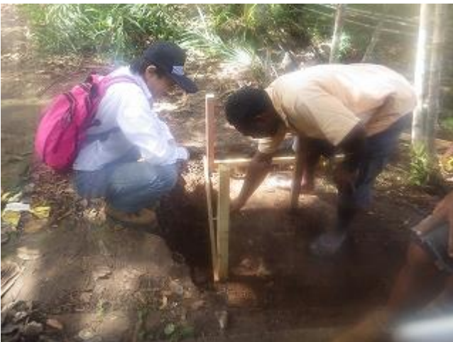
Photo 3: Mr. Imai of JICA inspecting the work for IC complex (VNP).
