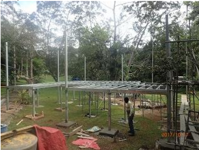
Photo 9: The construction of the new information center with steel posts and beams (VNP).
