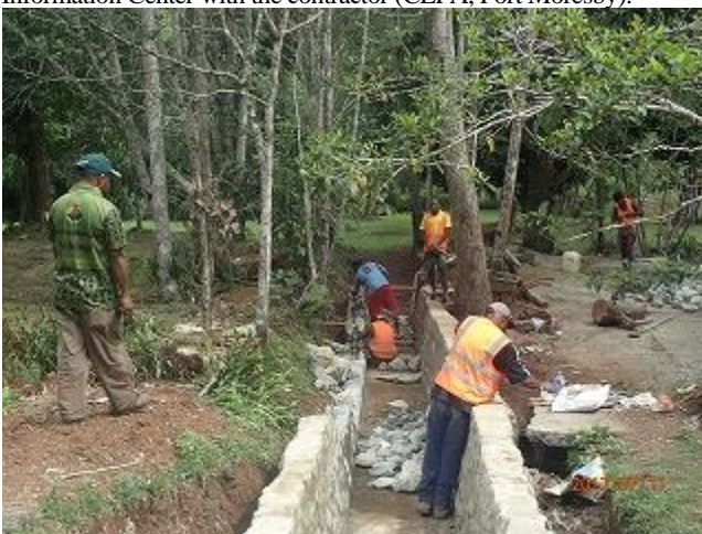
Photo 11: Local construction contractor, repairing the drainage of parking area in Varirata National Park (VNP).
