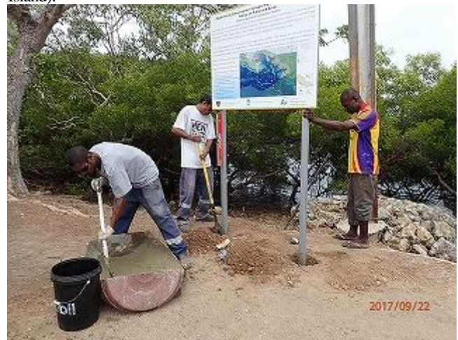
Photo 22: Local contractor installing signboards of CEPA-JICA marine project at Tahira (Tahira).
