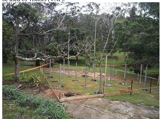
Photo 6: New information center was surveyed and pit and column were installed (VNP).
