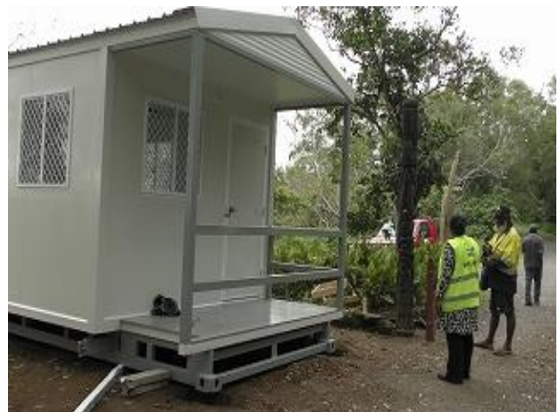
Photo 6: New tall gate house was established at the entrance of Varirata National Park (VNP).
