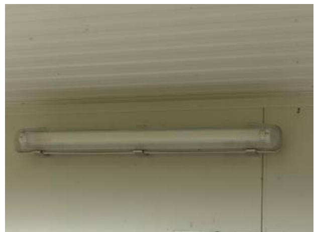
Photo 6: Security light was installed at the front of the Tahira Marine Office (Tahira).
