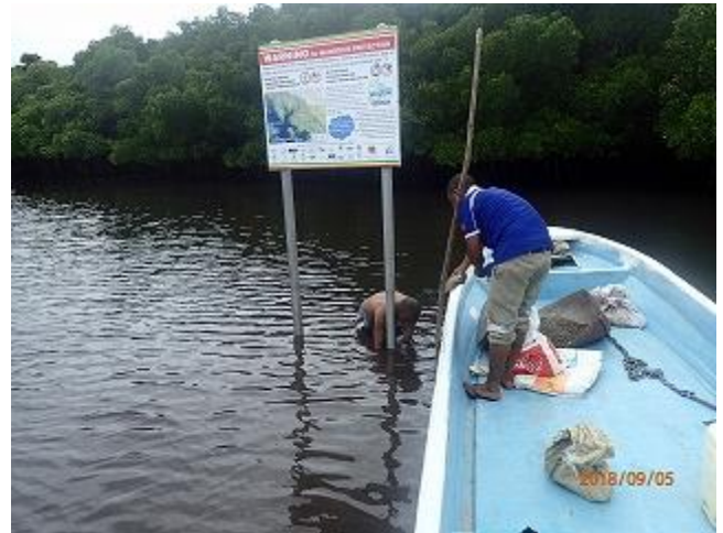
Photo 10: The installation of signboard for mangrove protection has been completed (Tahira).
