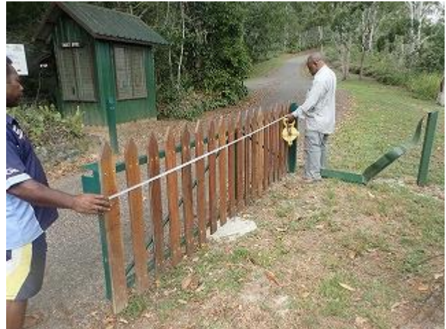
Photo 4: CEPA-JICA Team conducted monitoring work for renovated park facilities (VNP).
