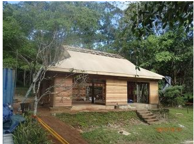
Photo 8: The renovation of the existing information center is ongoing. Photo showing side view (VNP).
