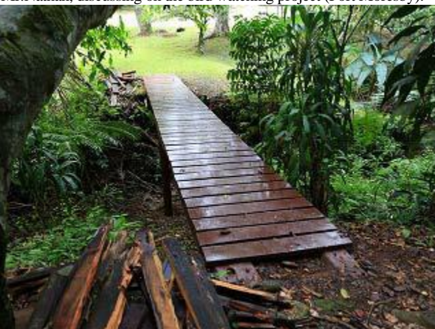
Photo 5: A photo of the wood bridge at the main picnic site of VNP, after renovation work by the Project (VNP).
