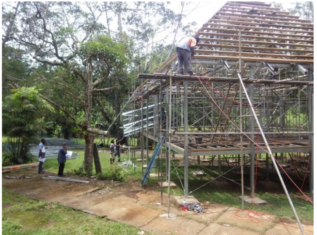
Photo 4: CEPA-JICA Project team inspecting the construction of the new IC (VNP).
