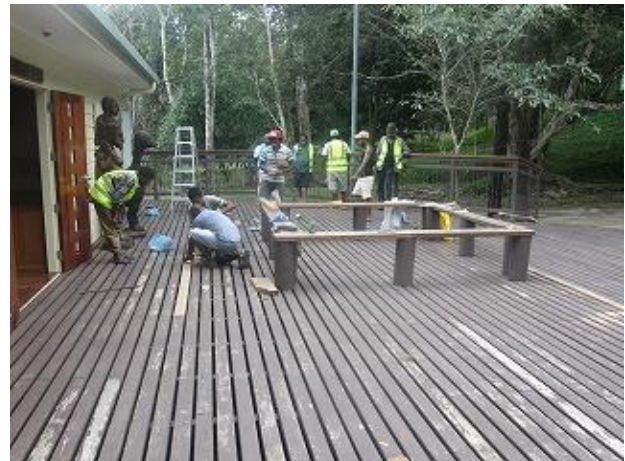
Photo 4: CEPA-JICA project team, repairing wood decking at Varirata National Park (VNP).
