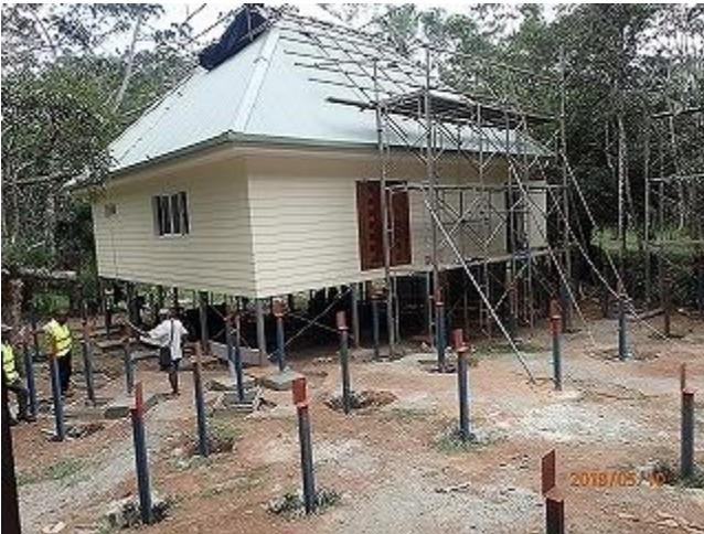
Photo 3: The installation of steel posts for wood decking were ongoing (VNP).
