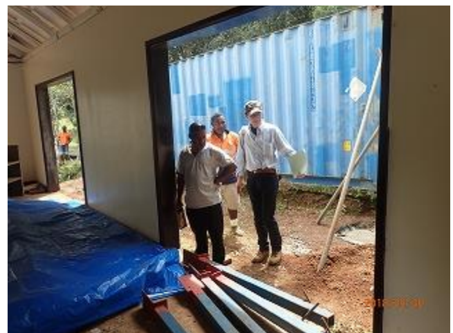
Photo 6: Mr. Imai of JICA checking work progress of renovated old information center (VNP).
