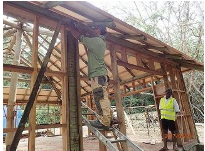
Photo 8: Auditorium is being renovated by local contractor (VNP).
