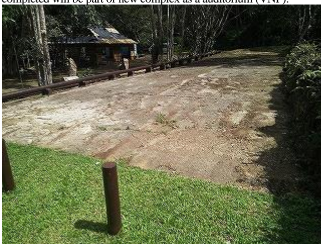
Photo 5: Renovated parking areas with new car stop piles recently installed (VNP).
