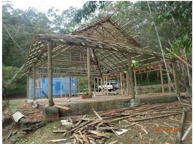
Photo 4: Roof repairing work is progressing for renovation of Old Information Center (VNP).
