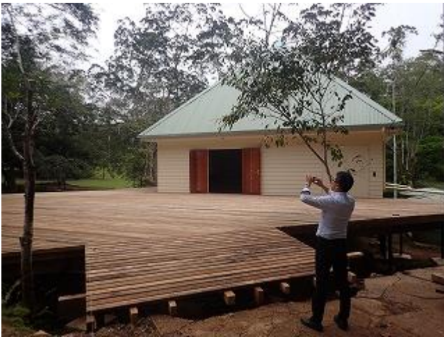
Photo 1: Mr. Hoshiai of JICA inspecting wood deck installation work for Information Center Complex (VNP).
