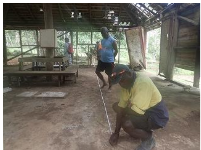
Photo 6: Local construction company has conducted a field survey for proposing renovation of the Information Center. (VNP).
