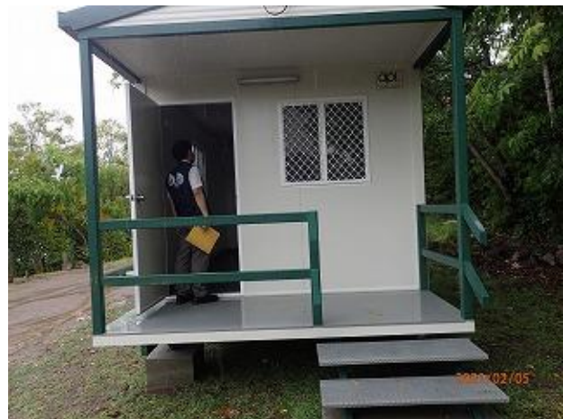
Photo 10: Mr. Asano of JICA, inspecting marine station office installed by API at Tahira (Tahira).
