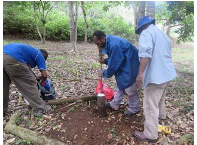
Photo 4: Work for distance pile installation. (VNP).
