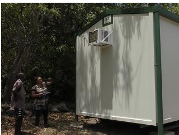
Photo 11: CEPA-JICA project team, checking the condition of the Tahira marine office (Tahira).
