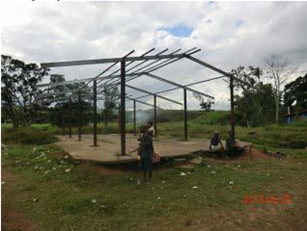
Photo 3: Sogeri Local Market construction site (Koiari LLG).
