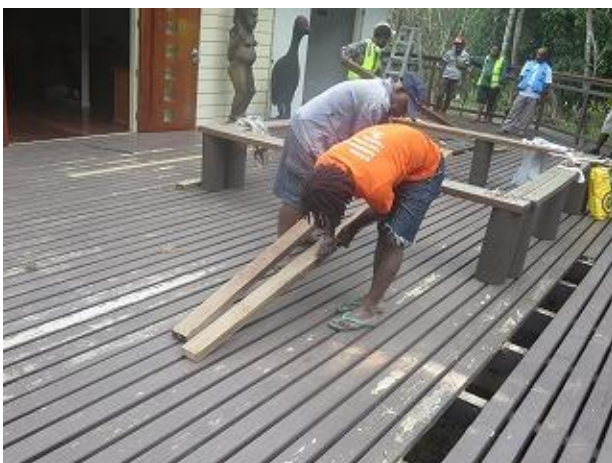
Photo 5: Mr. Tati of park staff, sanding woods to repair wood decking at Varirata National Park (VNP).
