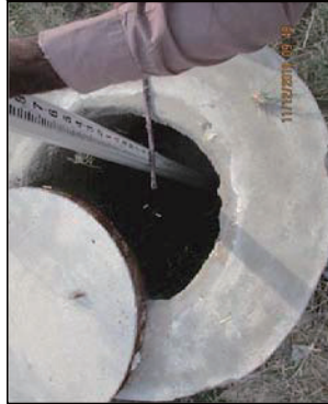
Measurement of depth of manhole
