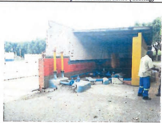
Photo-6 Pipe Fixing Training Yard of eThekweni Metro (KZN)
