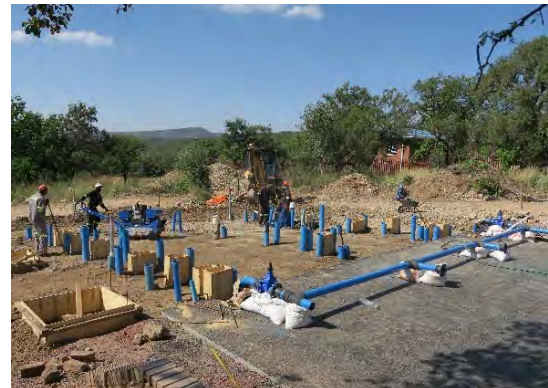
Photo-104 Yard Construction (after Backfill)
