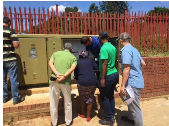
Photo-44 Electricity Inspection for Training Yard
