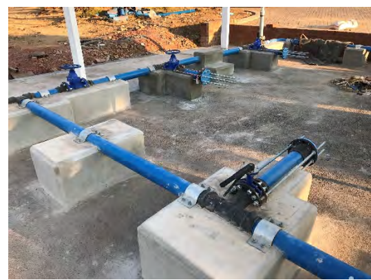
Photo-108 Training Yard (Pipe Connection Training Area)
