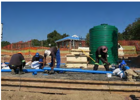
Photo-103 Yard Construction (uPVC Pipe Laying)
