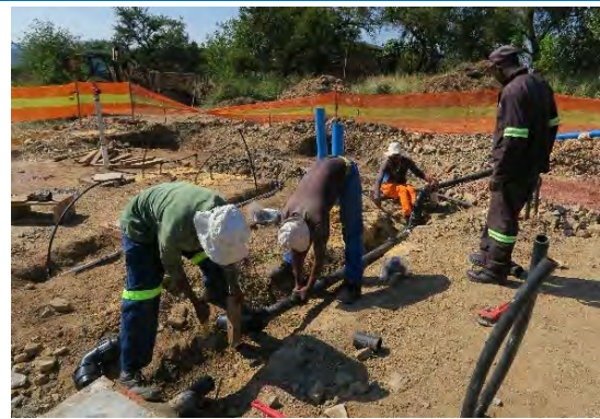
Photo-102 Yard Construction (HDPE Pipe Laying)
