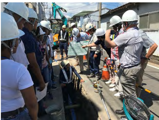
Photo-123 The 2 nd Training in Japan (Construction Site)
