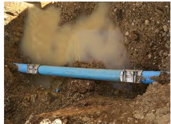
Photo-38 Site Visit (Leak Repair by Tshwane)
