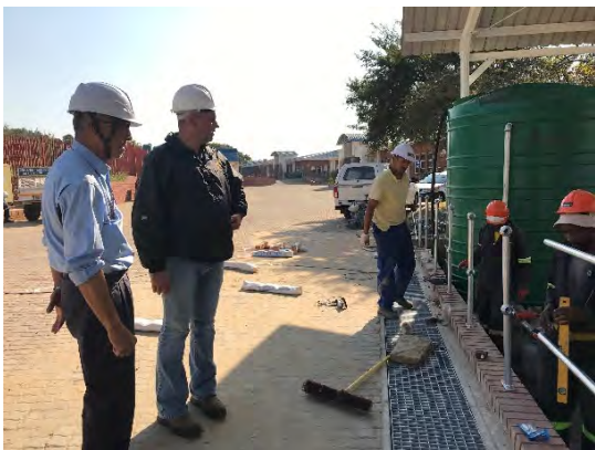
Photo-107 Supervision of Yard Construction
