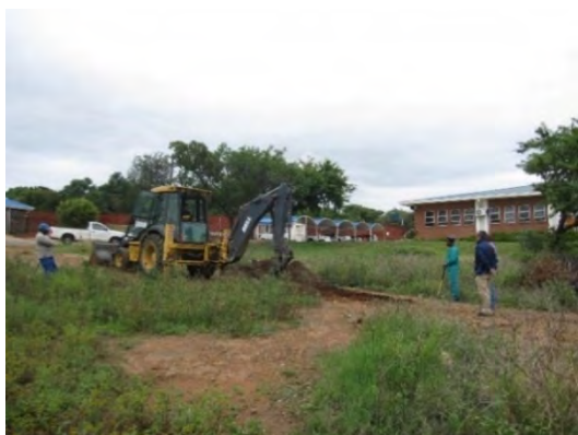
Photo-27 Test Excavation at Training Yard
