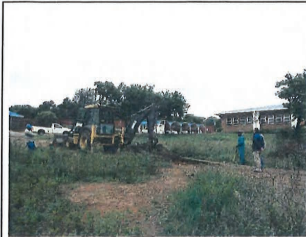
Photo-1 Confirmation of Underground Pipe at Candidate Location of Training Yard in IBTC
