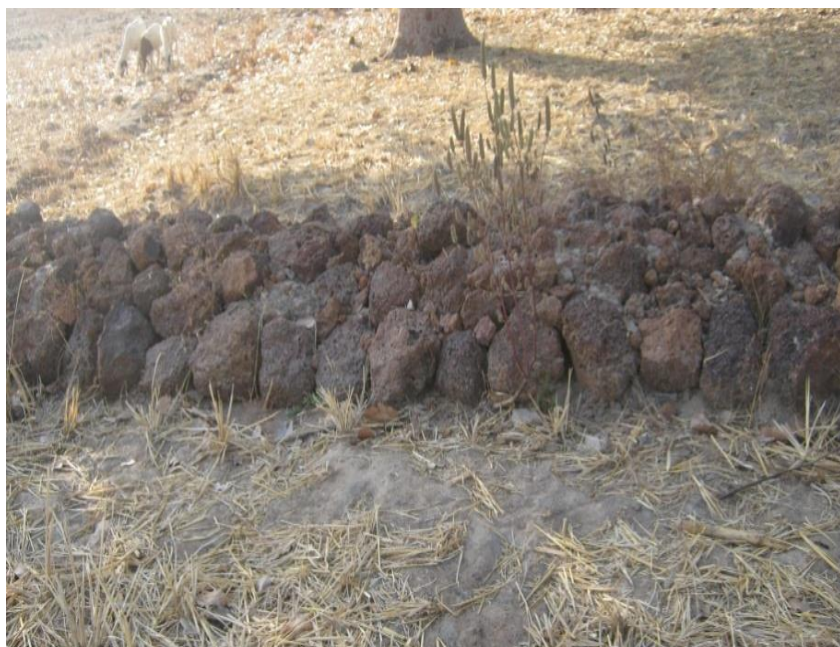
Stone Bunding (across the water flow direction)
