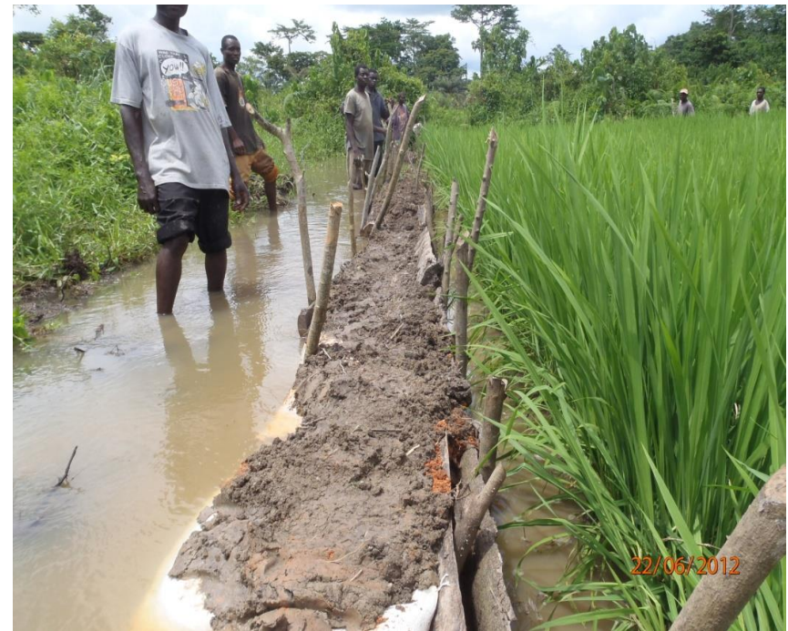
Using Sand bags with wooden materials
