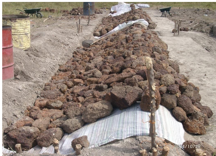
Combined earth & Stone Bunding with impermeable sheet
