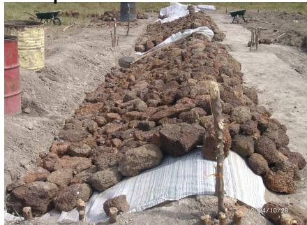
Combined earth & Stone Bunding with impermeable sheet
