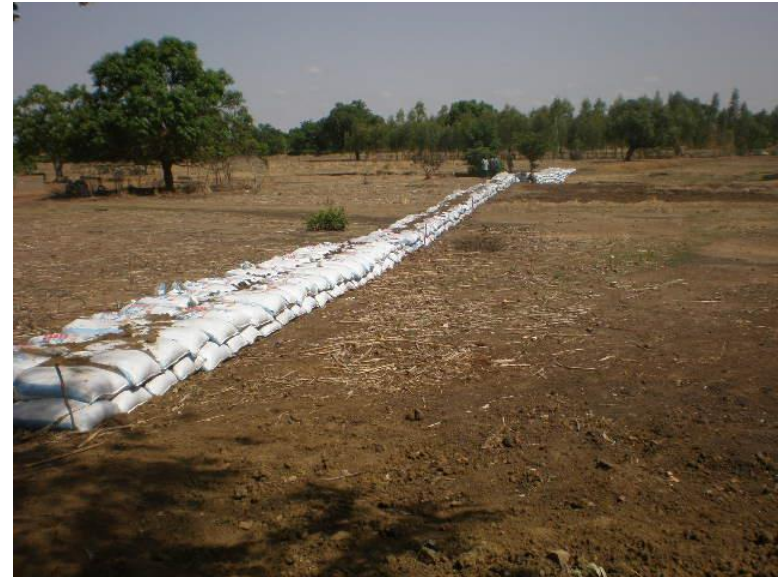
Bunds with sand bags
