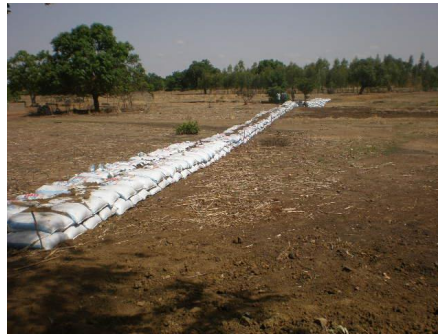
Bunds with sand bags
