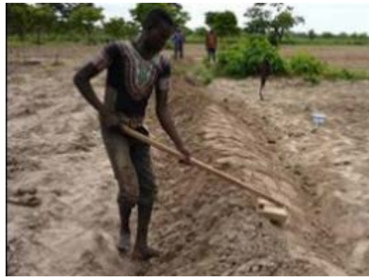
Picture 26 Bund Construction (Central Gonja)
