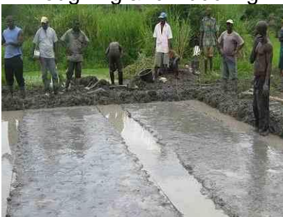
Completed wet nursery bed
