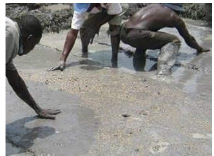
Covering by soil
