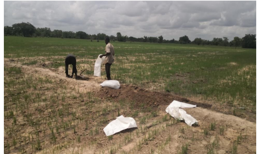
Fig. 7 Karaga district Use sand bags to reinforce the bund.
