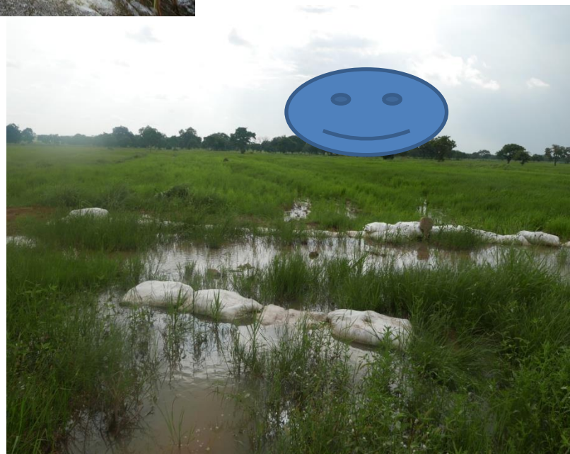
Bund protection With sand bags Savelugu
