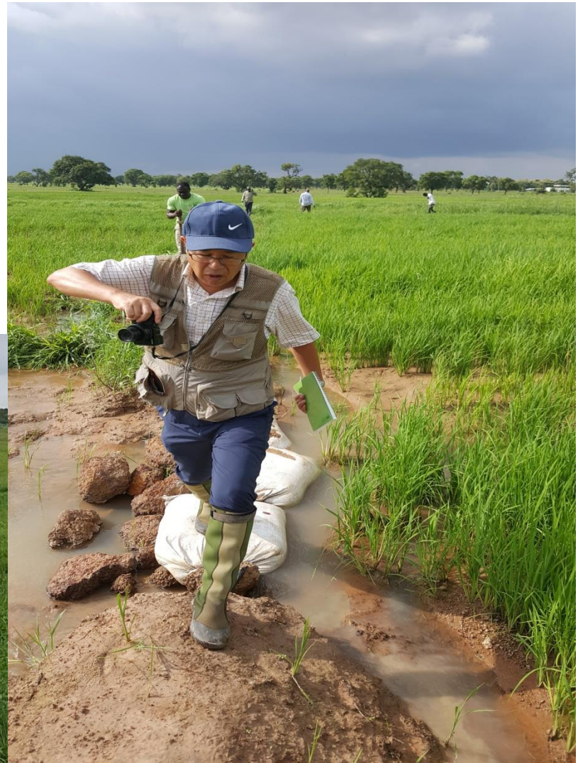
Using Sand bags/ stones for bund maintenance (Savelugu district)
