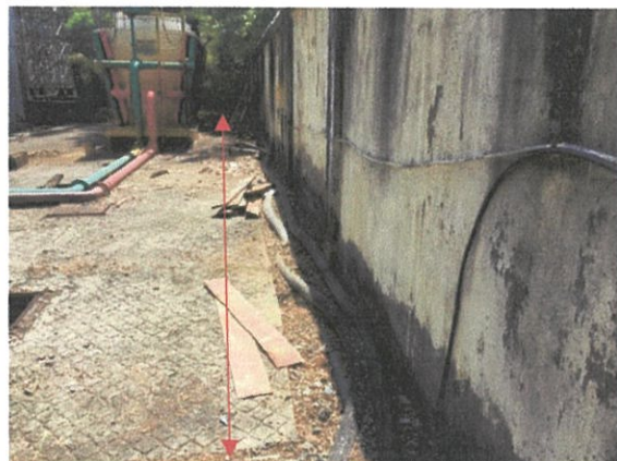
New cable trench route
