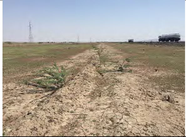
8. Old trace of Excavation for OFC.
