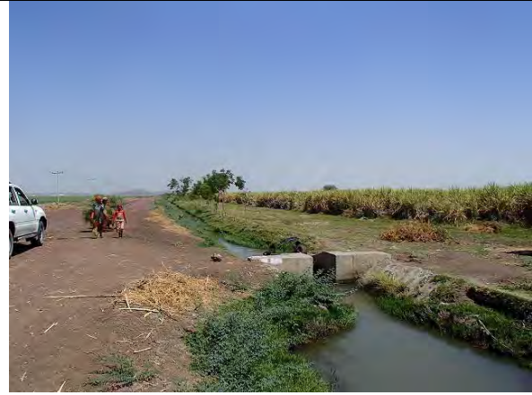
10. SC1-5. Canal has 2m in width and is excavated ditch without surface treatment.
