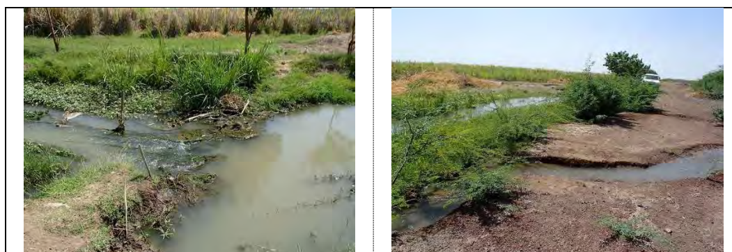
Figure A11.3.4 Sedimentation of Debris (left) and Erosion by Overflow (right) in SC1-5
