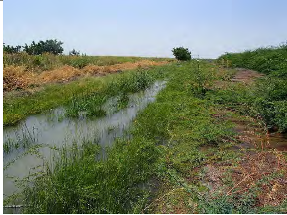
13. SC1-5. Due to depositing debris and waterweed, overflow has occurred.
