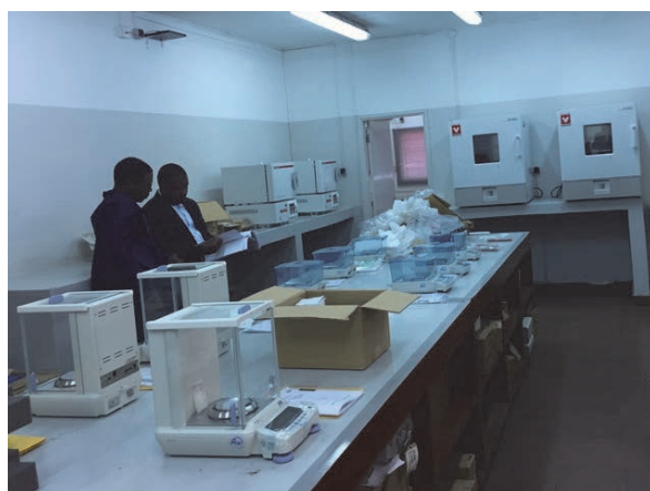
Photo 2.3-15 Status of Installation for the Donated Equipment
