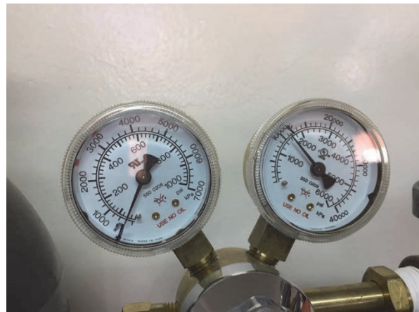
Photo 2.3-44 Decompressor Gauge (O 2 cylinder)
