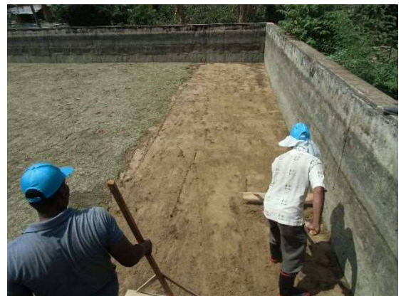
Figure 2-10 Sand Scraping Work by Using Wooden Scraper
