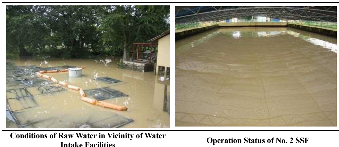
Photo 4-4 Continuous Operation in No. 2 SSF
