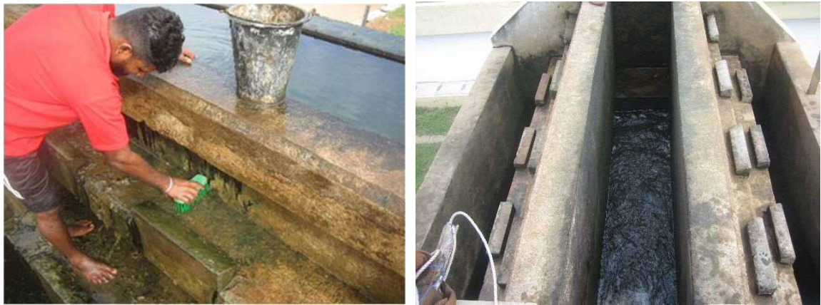
Figure 2-7 Cleaning Work of Aerator
