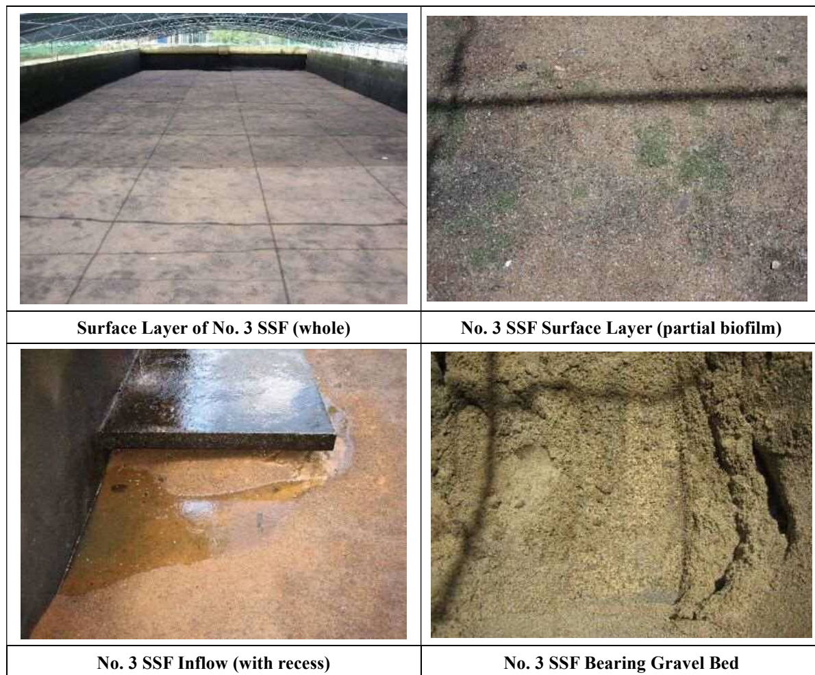
Photo 3-12 Filter Media Condition of No.3 SSF
