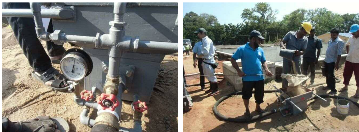
Figure 2-14 Pressure Gauge of Sand Ejector Unit (Left) and Throwing of Scraped Sand (Right)
