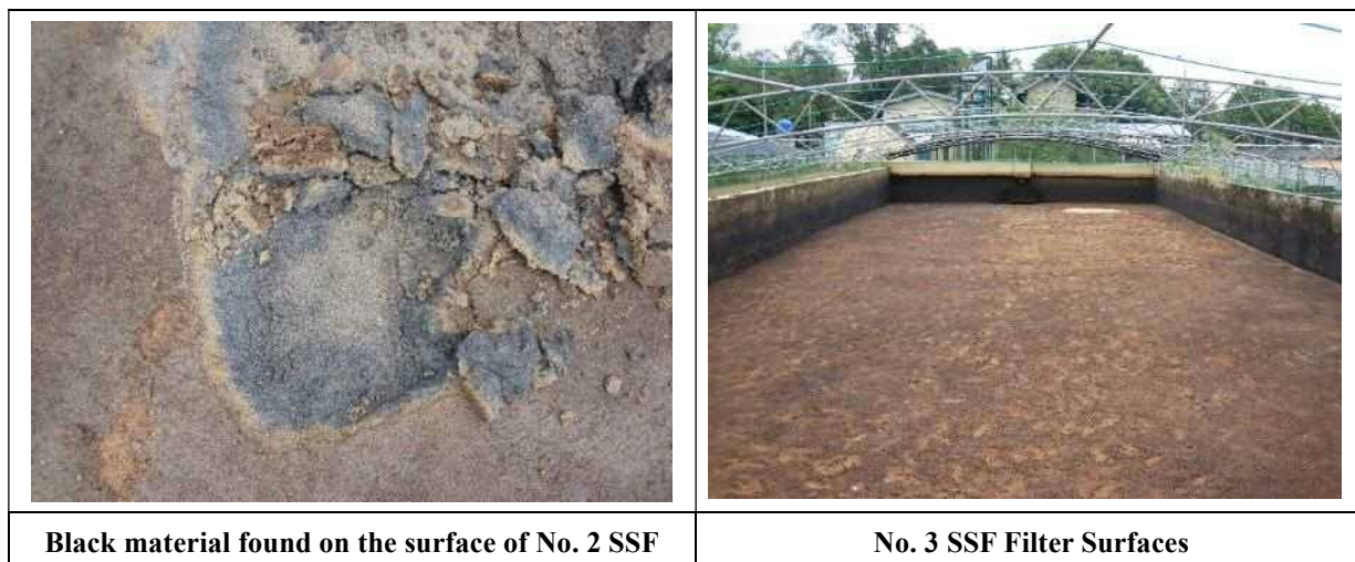
Photo 3-5 Detail Condition of No. 2 and No. 3 SSF
