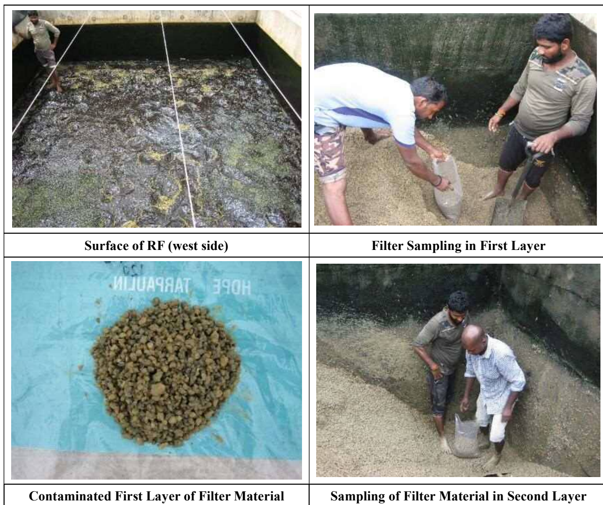
Photo 3-10 Investigation in RF (West)
