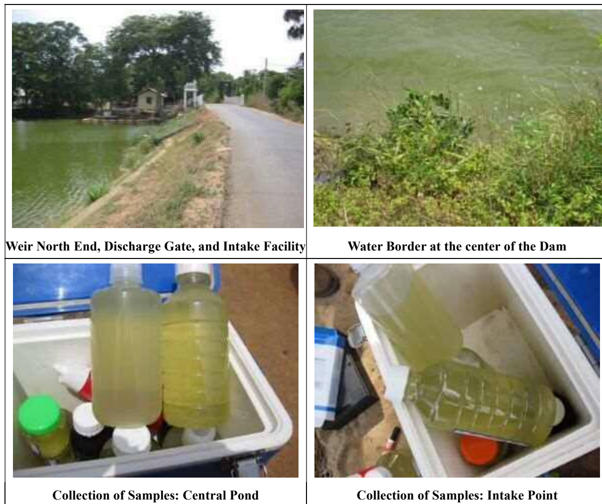
Photo 3-2 Status of Dry Aru Reservoir (Dry Season)
