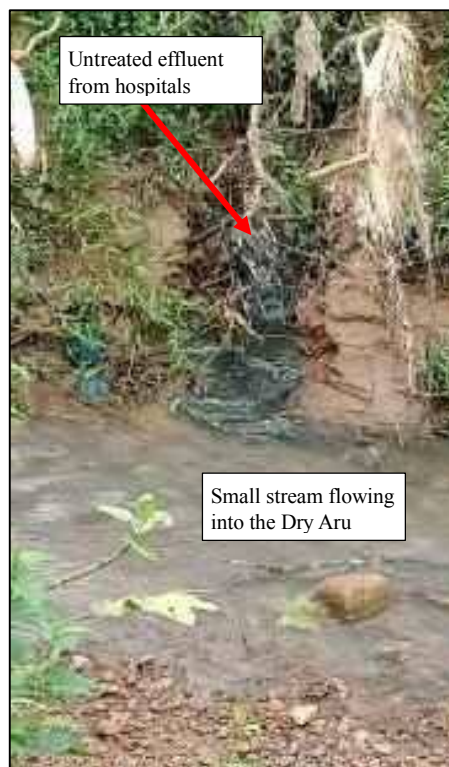
Photo 5-4 Outflow of Wastewater
