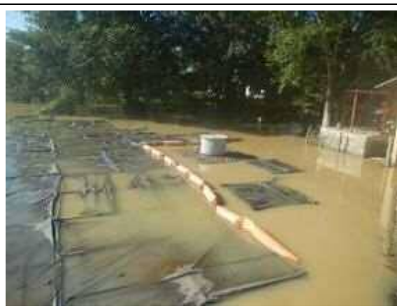
Photo 4-2 Current status of Dry Aru reservoirs (Rainy Season)
