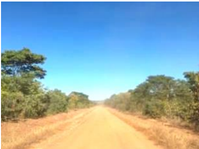
Unpaved road to Chikumbiro FB.
