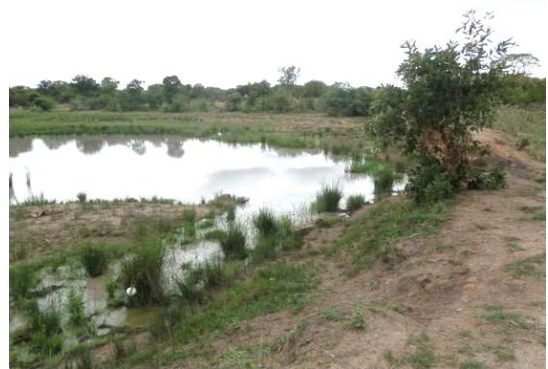
Community earth dam at Katumbi site in the FB
