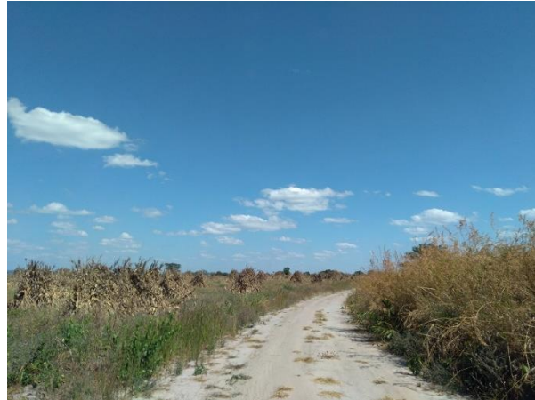
Surface conditions of an access road in Luena. The road width is approximately three to four meters, and it is not paved.
