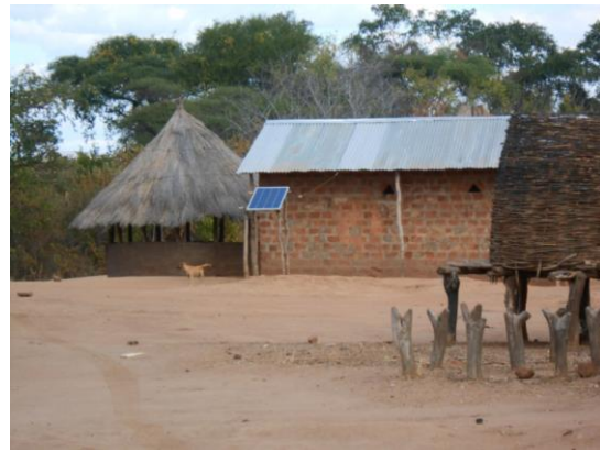
Existing residence with a solar panel (center) and crop storage (right)
