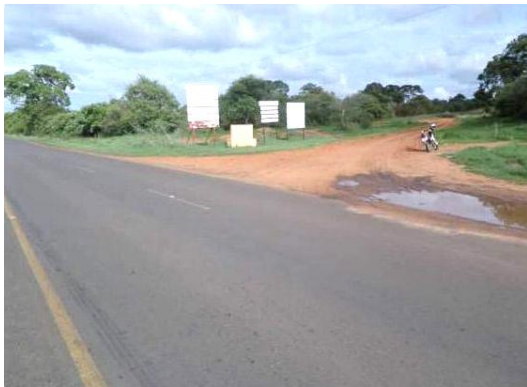
The trunk road (Livingstone-Kazungula Road) and its junction to Musokotwane FB. The FB is 60 km from this point.
