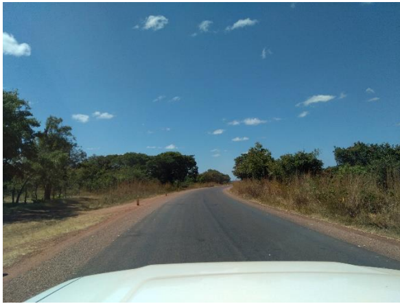
Road surface conditions of the two-lane trunk road north of Luena FB (from Kawambwa town to Muporokoso)
