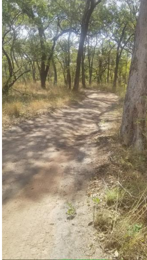
Road in Luswishi FB: Too narrow for large vehicles to pass through
