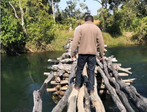
Crossing point of the Lwangwa River from the northern boundary of Kalungwishi FB
