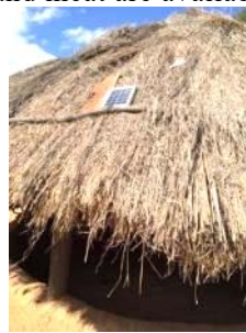
Solar panel on the roof of the meeting place in the FB. Farmers use electricity to charge their mobile phones.
