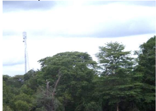
Communications tower at the Makunka site 17 km away from the FB
