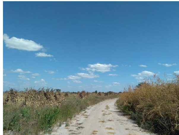
Surface conditions of an access road in Luena. The road width is approximately three to four meters, and it is not paved.
