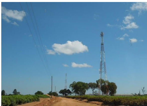
Communication towers along an access road in Luena FB. The ZAFFICO Tea plantation can be seen on both sides of the road.
