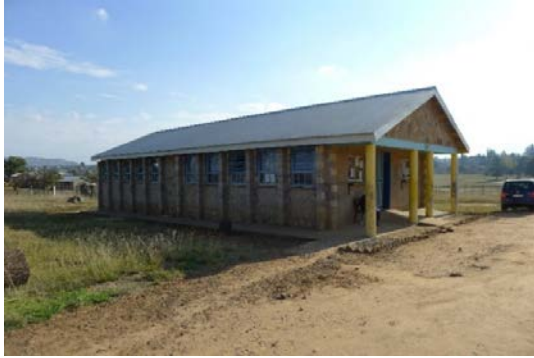
General View: South side of Administration building
