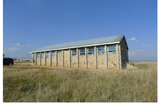
General View: North side of Administration building
