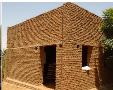
Construction of generator house
