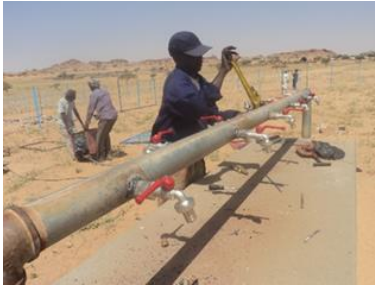
Replacing the broken taps with a new one.
