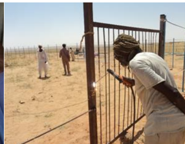
Installation of fence around water yard.
