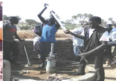
Rehabilitation of hand pumps by community residents (total 33 pumps were repaired under supervision of SWC)
