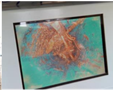
Inside of well captured by special scope. Tree root invaded and trash is also found in borehole.
