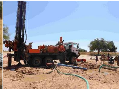
Drilling of borehole by contractor
