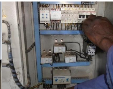
Setting-up control panel.
