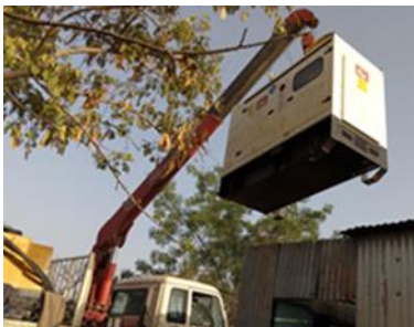
Replacing the old generator with a new one.
