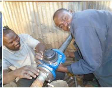
Installing a water meter to measure water usage.
