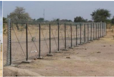
Fencing of water yard
