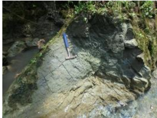
Photo 1.2-6 Siltstone is stiffened but easy to be stabbed with a pick of hammer. Kneading rock on hands become easily liquefaction. Shrinkage cracks due to dry are found on outcrop surfaces.
