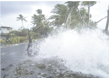
Fig. 2. Wave Overtopping at Hinterland. (Before the Project)
