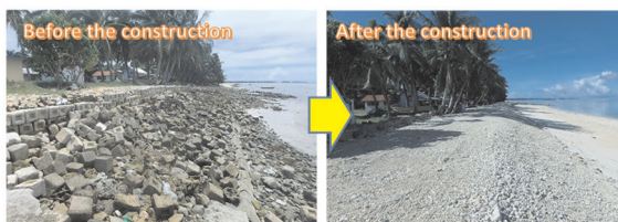
Fig. 2. Before and after the Project (gravel beach nourishment).
