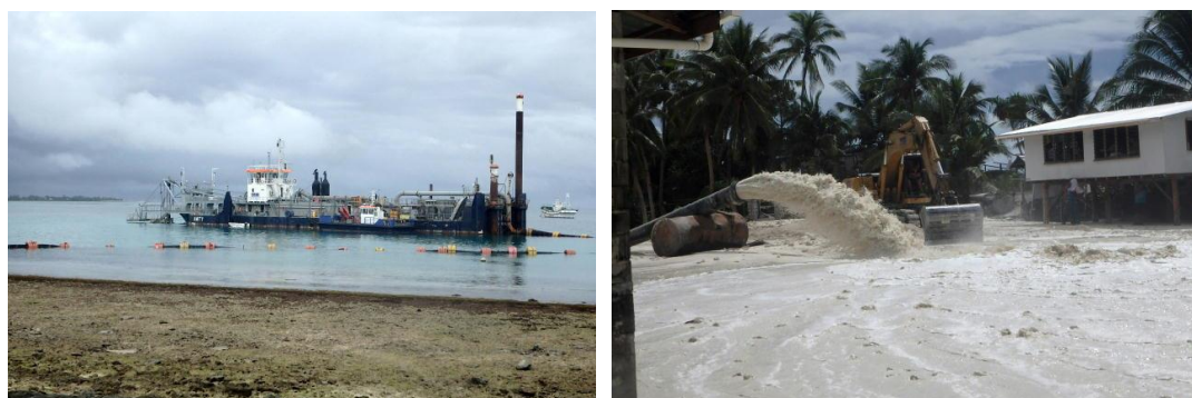
Figure 17.3.6 Sand Dredging Activity (Borrow Pit Project by NZ Aid)
