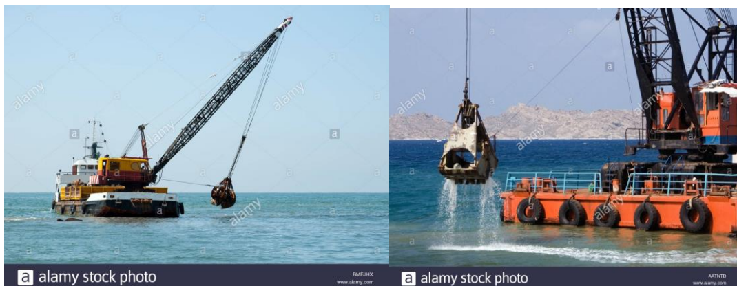
Figure 17.3.3 Example for Crane Barge Attached with Clam Shell Bucket)
