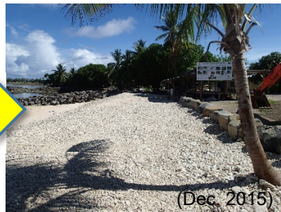
Beach nourishment completed
