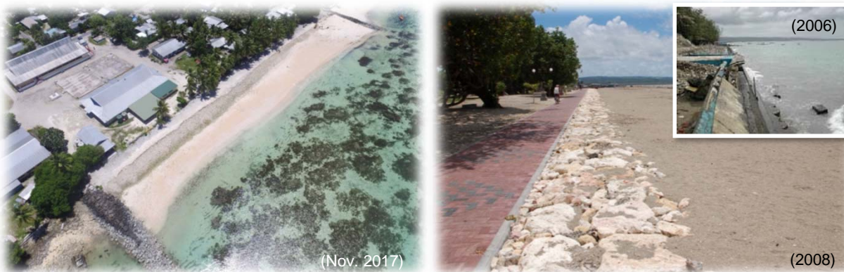
(e.g. 3) Nourishment with groins (Tuvalu) (e.g. 4) Nourishment with backshore revetment (Bali)
