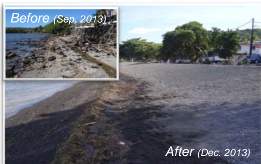
ex.3 Dynamically Stable Beach Method (Only gravel filling) - Mauritius -
