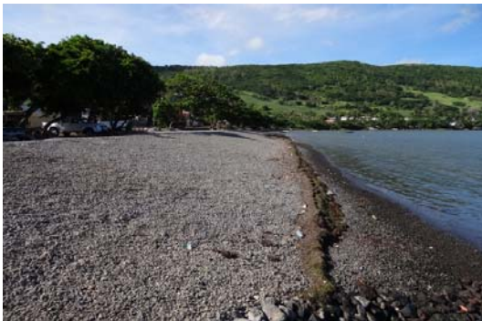
Just after the Construction (Dec. 2013)
