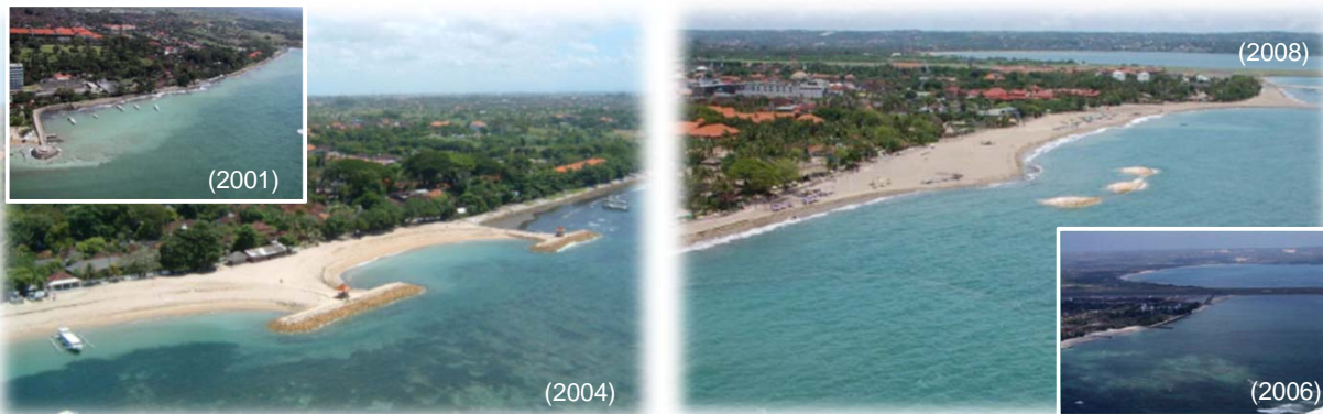
(e.g. 1) Nourishment with groins, headlands (Bali) (e.g. 2) Nourishment with offshore breakwaters (Bali)
