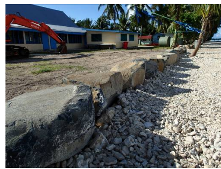
Figure 9.5.7 Armor Stones for Backshore Stone
