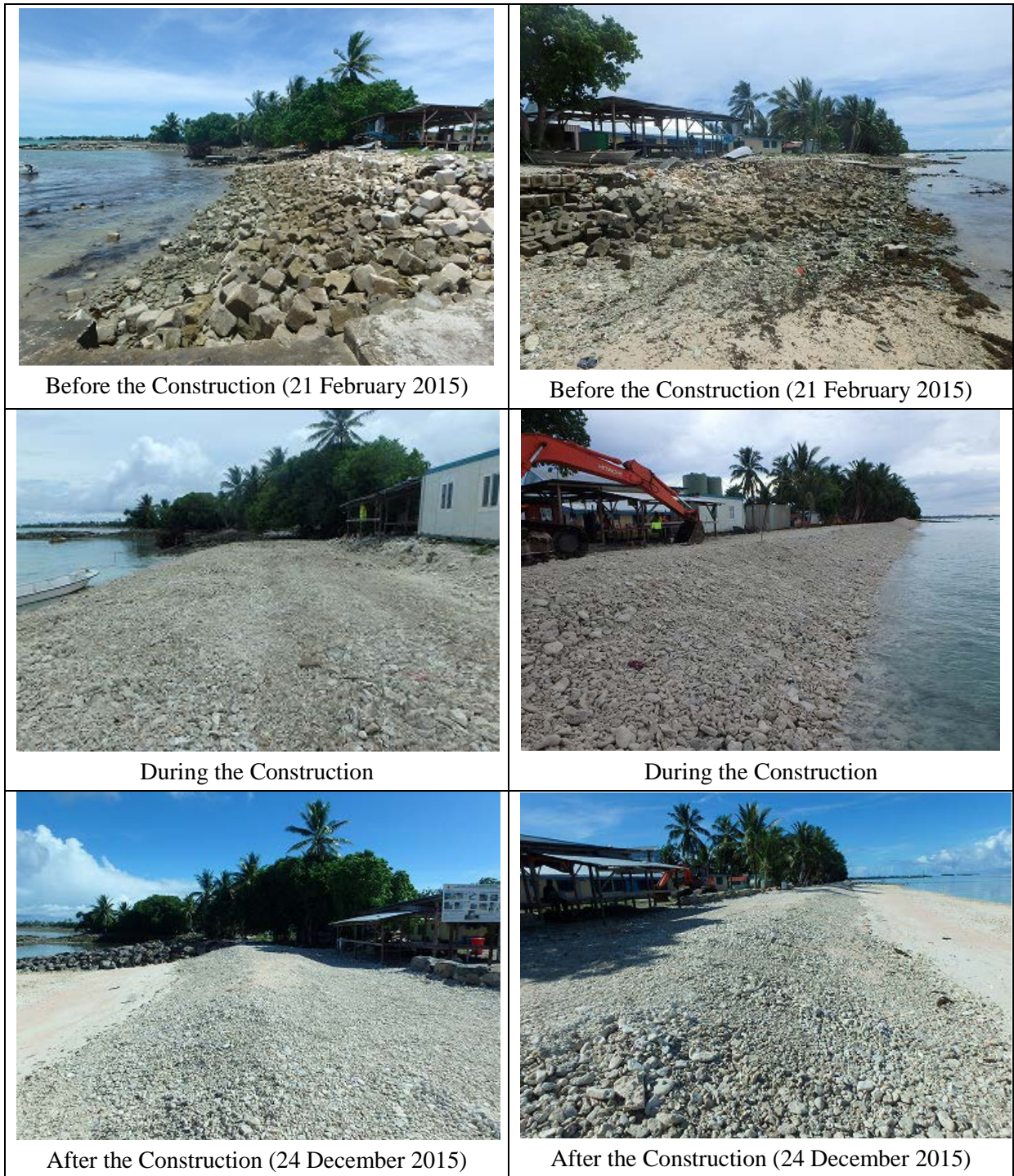
Figure 9.8.1 Comparison of Photos Before, During, and After the Construction
