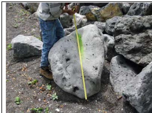
Figure 9.4.1 Inspection of Armor Stone in Taveuni Island, Fiji
