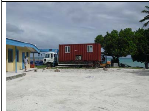
Figure 9.4.3 Temporary Site Office
