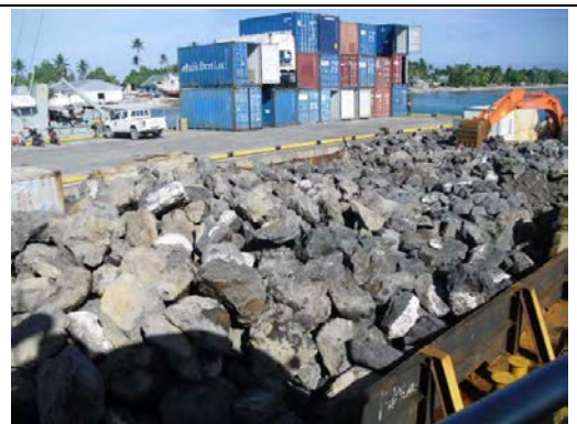
Figure 9.4.4 Transportation of Armor Stone and Equipment
