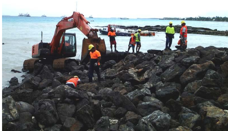
Figure 9.3.2 Groin Construction with Added Safety Measures
