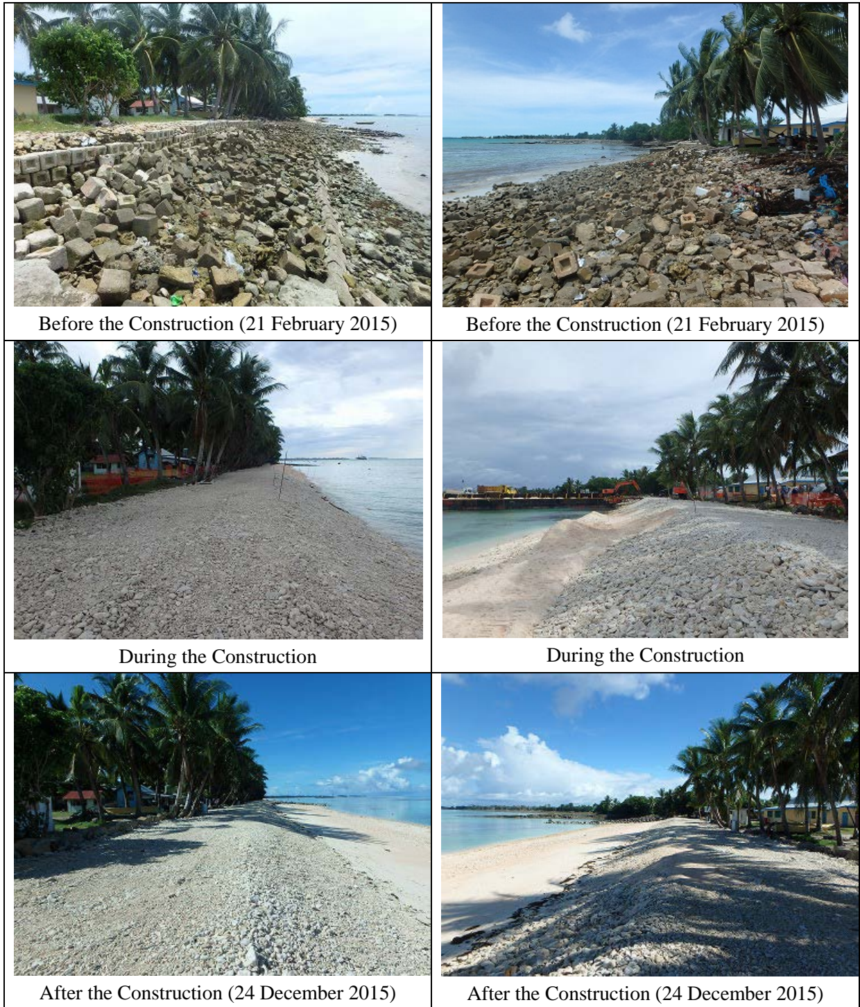
Figure 9.8.2 Comparison of Photos Before, During, and After the Construction
