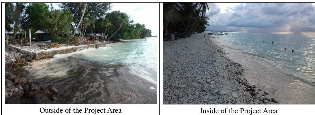
Figure 9.8.5 Comparison of Wave Condition Inside and Outside of the Project Area during the King Tide (9 February 2016, 5:30 PM, +3.18 m from Tide Prediction)
