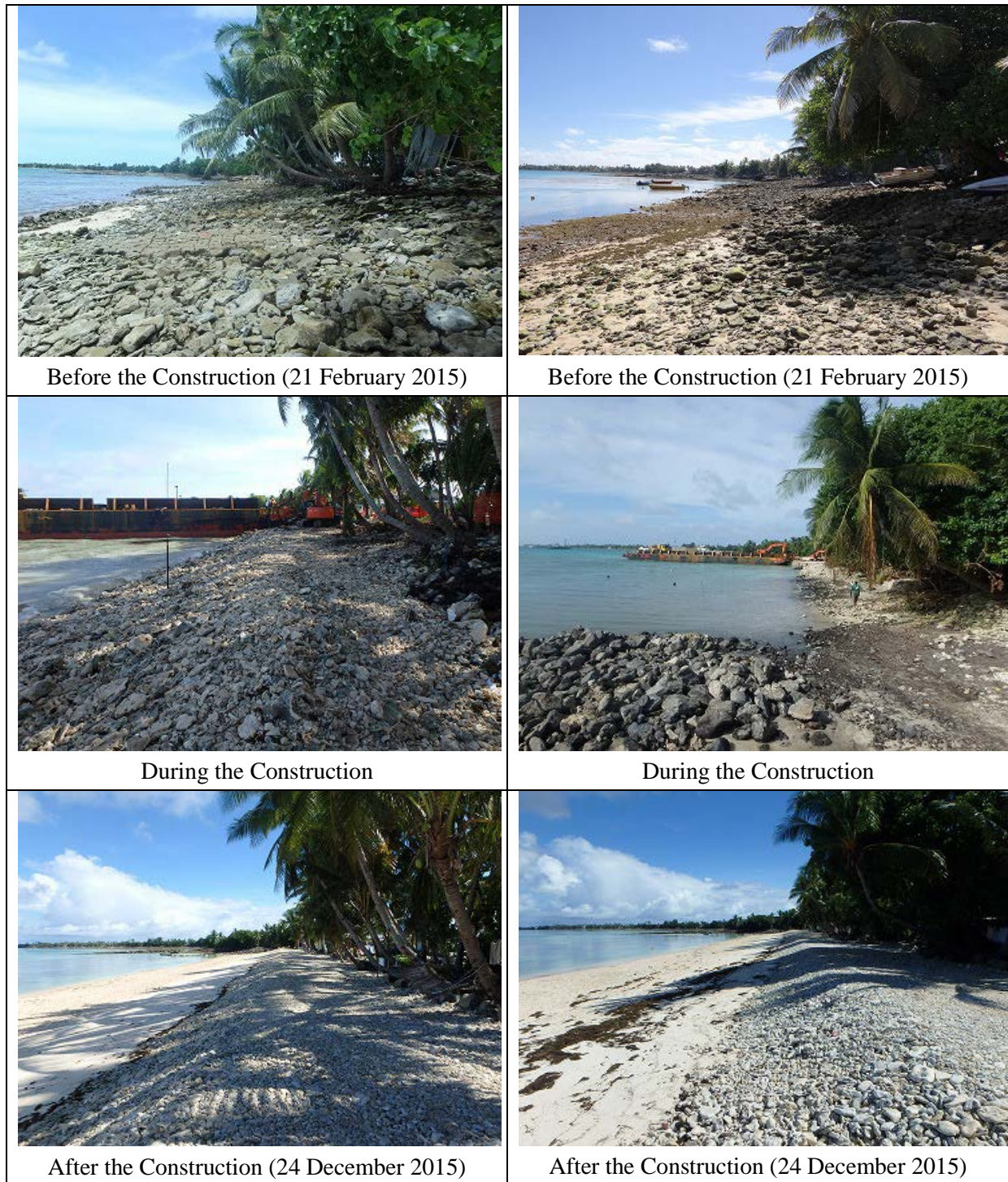
Figure 9.8.3 Comparison of Photos Before, During, and After the Construction
