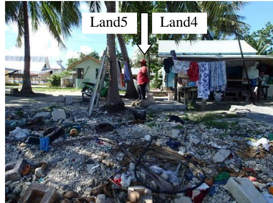
Boundary b/w Land 4 and 5 (Foundation)
