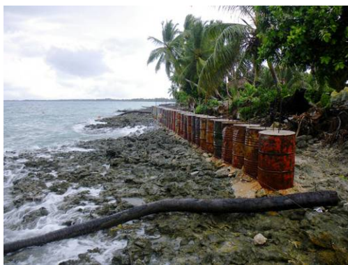
Figure 1.3.4 Barrier of Concrete in Oil Drum
