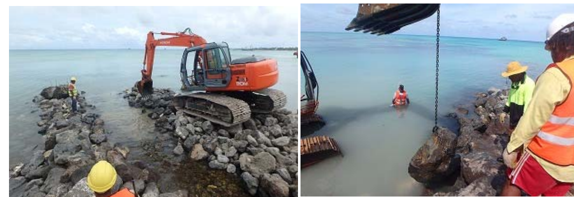
▲ Placement of Core Stones from Fiji ▲ Placement of Armor Rock from Fiji
