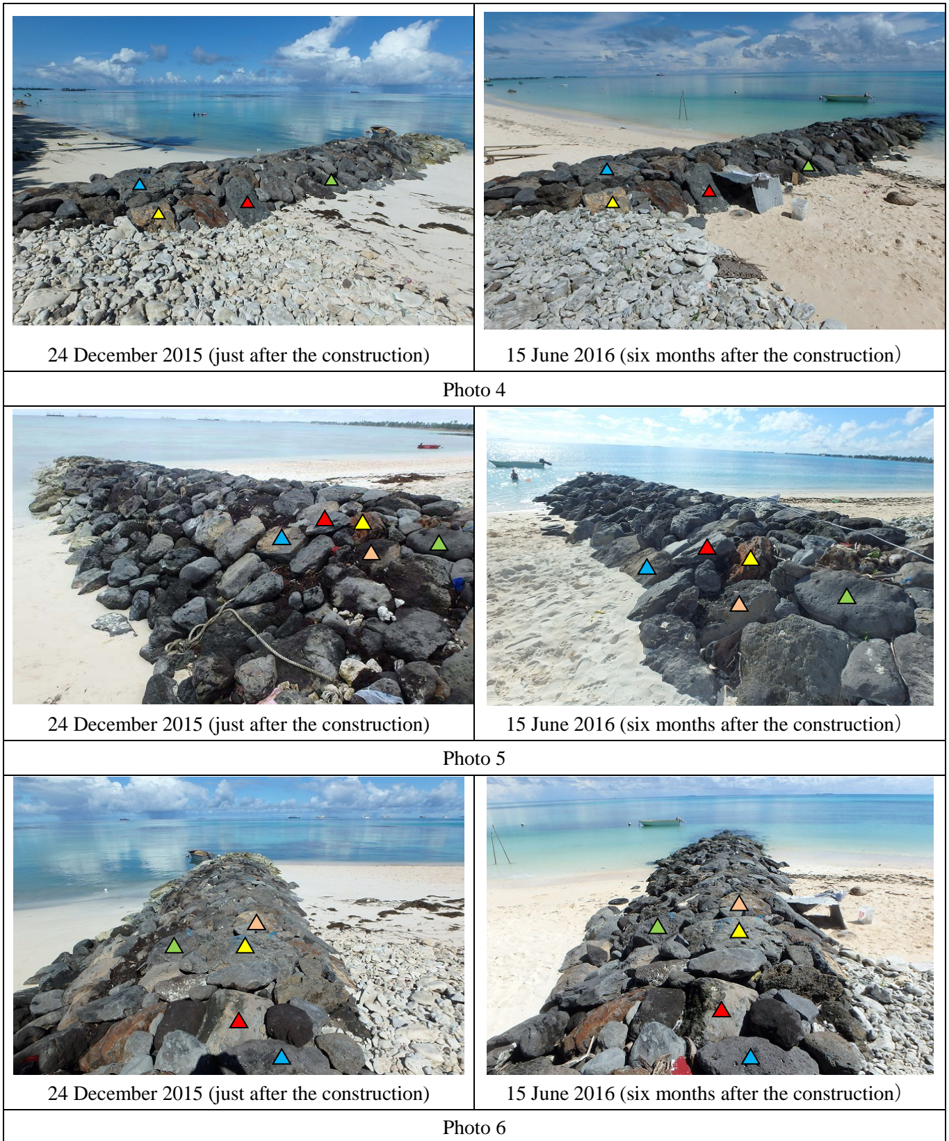
Figure 9.6.3 Comparison of the South Groin
