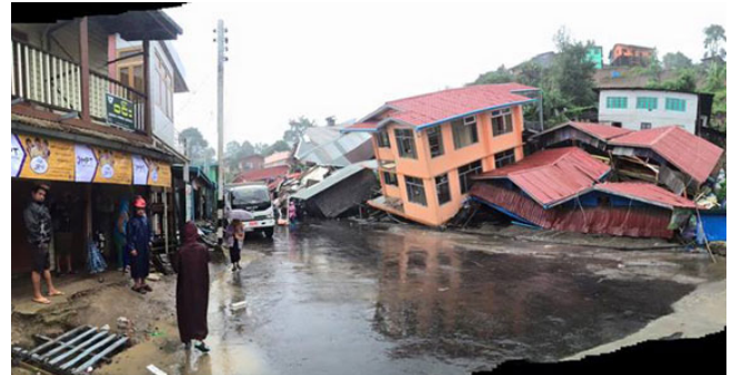
A mudslide in Hakha, the capital city of Chin State, destroyed several buildings. https://www.heavensfamily.org/urgent-need-in-myanmar/
