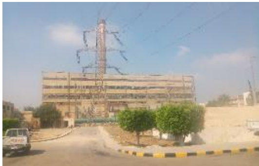
Investigation on the Talkha power plant
