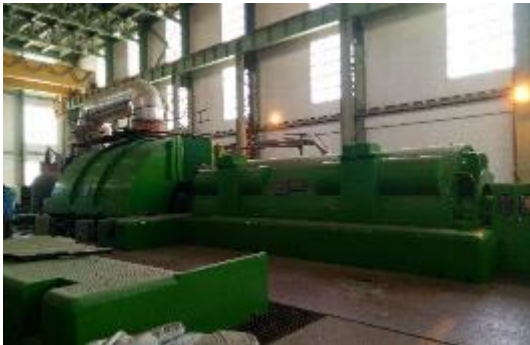
Investigation on the Assiut power plant
