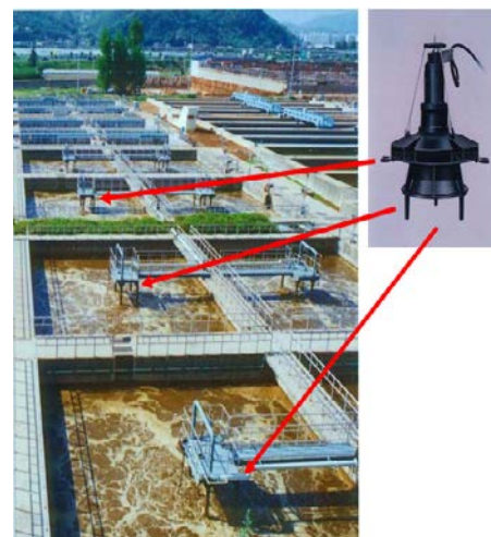
Figure 3.13 Energy Saving Type Diffuser (Aerator Type)
