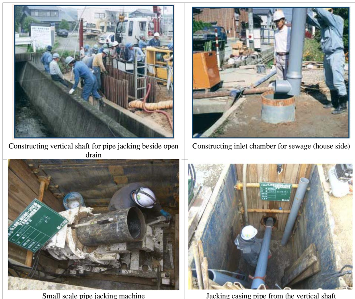
Figure 2.4 Photos of Small Scale Pipe Jacking for House Connection
