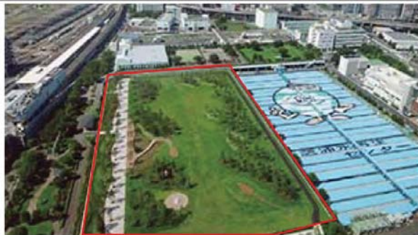
Underground Plant (Red Area)
