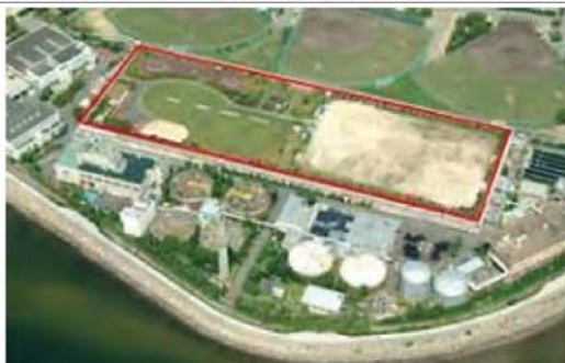
Underground Plant (Red Area)
