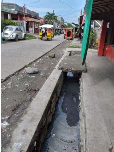
Agdao Dist. Brgy Paciano Bangoy: street and drain
