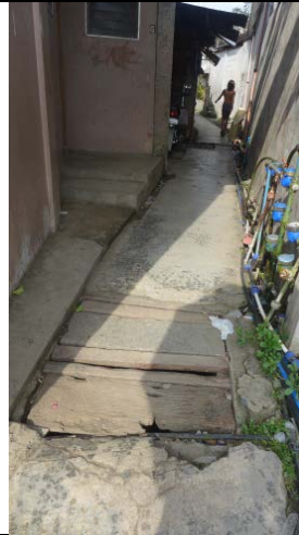
Brgy. 1-A residential area (covered drain)
