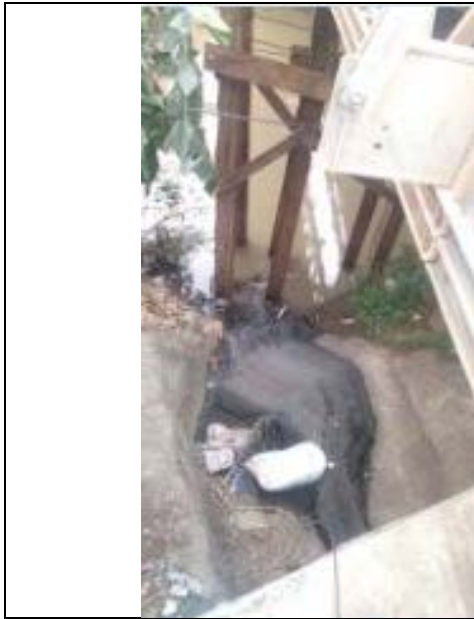
Area C Brgy Talomo: Talomo Bridge on Talomo River with outfall
