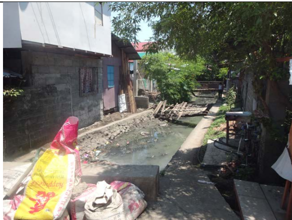
Brgy 76A Bucana: Open drain towards Davao River
