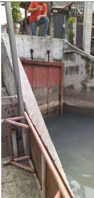
Brgy 2-A: Gate at exist of drain
