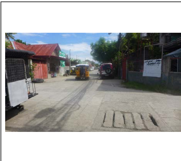
Agdao Dist. Brgy Centro San Juan: street with underground drain
