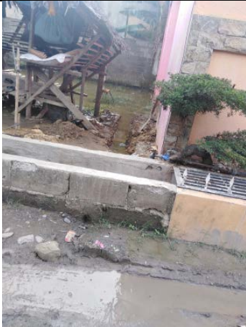
Area C Brgy Bago Aplaya: street with new drain
