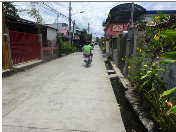
Brgy. Lapu-Lapu: street with open drain
