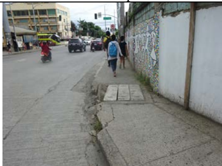
Area B: Brgy. Buhangin (covered side drain)
