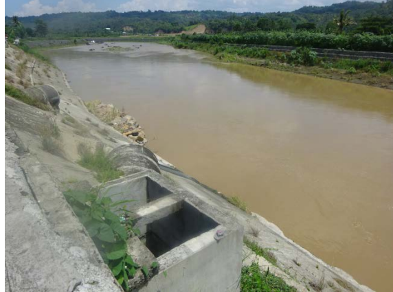
Brgy Tigatto: outlet from open channel to Davao River
