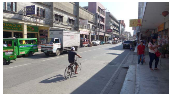
Brgy 27-C: Street in commercial area with covered side drain
