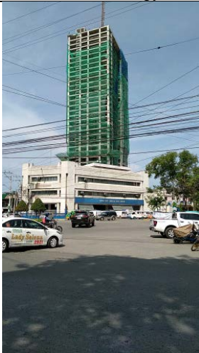
Brgy 4A: large apartment under construction
