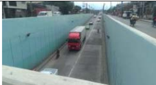
Area B: Brgy. Buhangin (under path)
