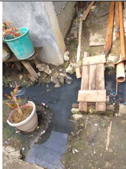
Brgy. Vicente Duterte drain
