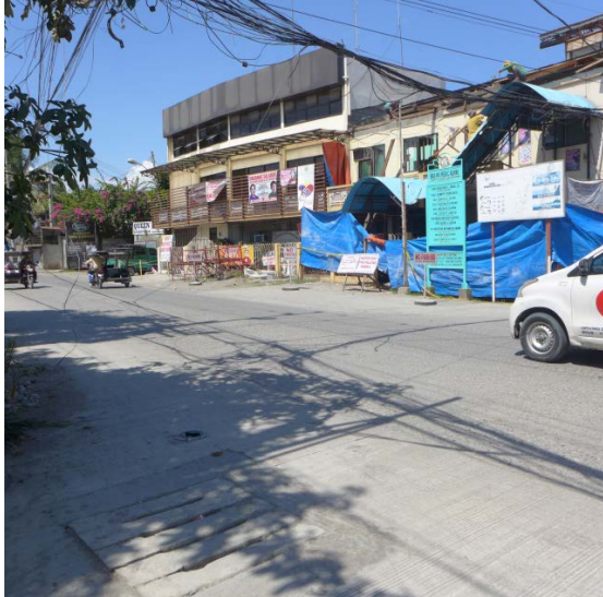
Brgy. Wilfred Aquino: road with underground drain
