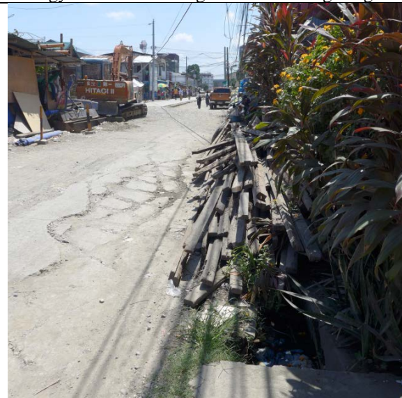
Brgy. Ubalde: Road with open drain
