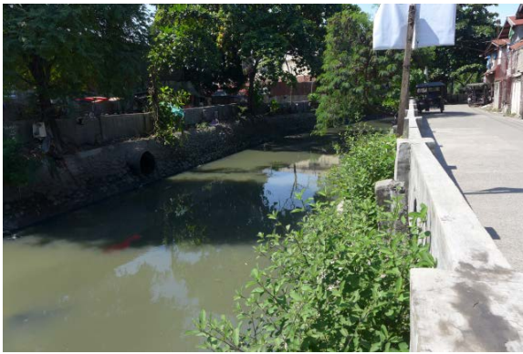
Dacudao Creek with outlet (Brgy Leon Garcia)
