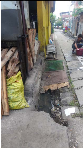
Brgy 32-D Drain
