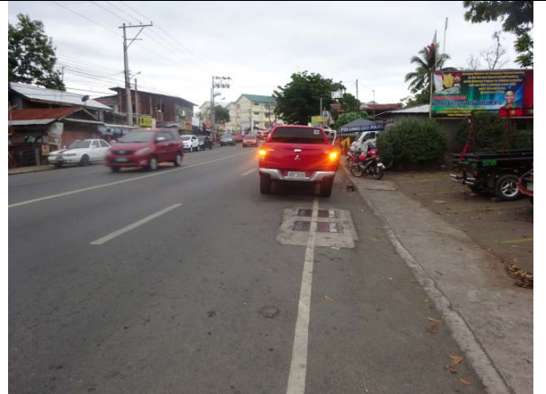
Area E: Brgy. Mintal (covered side drain)
