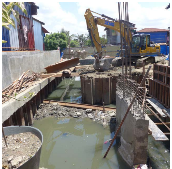
Pumping Station under Construction in Jerome Creek (Brgy Centro San Juan)
