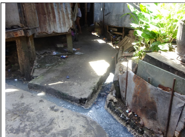
Photo 5.3.2. Narrow and Curving roads where Wastewater flows in Barangay Tomas Monte Verde in Area-A Agdao
