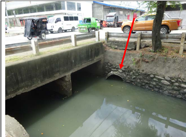
Photo 5.3.4 Submerged Outfall in Dacudao Creek
