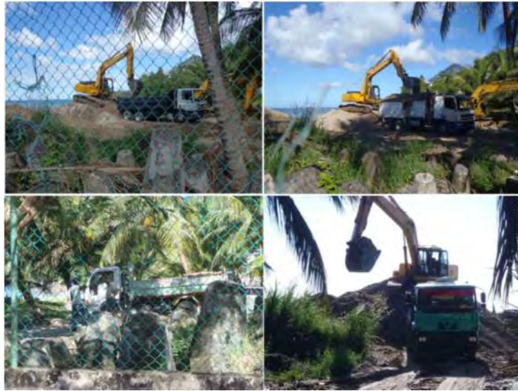
Photo 2-68 Transportation of dredged sand by truck (November 2017)
