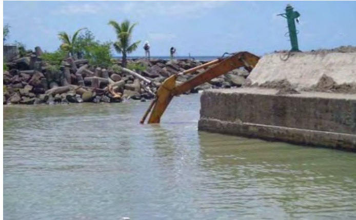
Photo 2-81 Dredging work by backhoe on August 21, 2018
