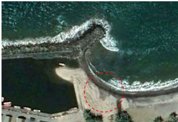
Photo 2-84 Trace of sandy beach excavation on March 24, 2018
