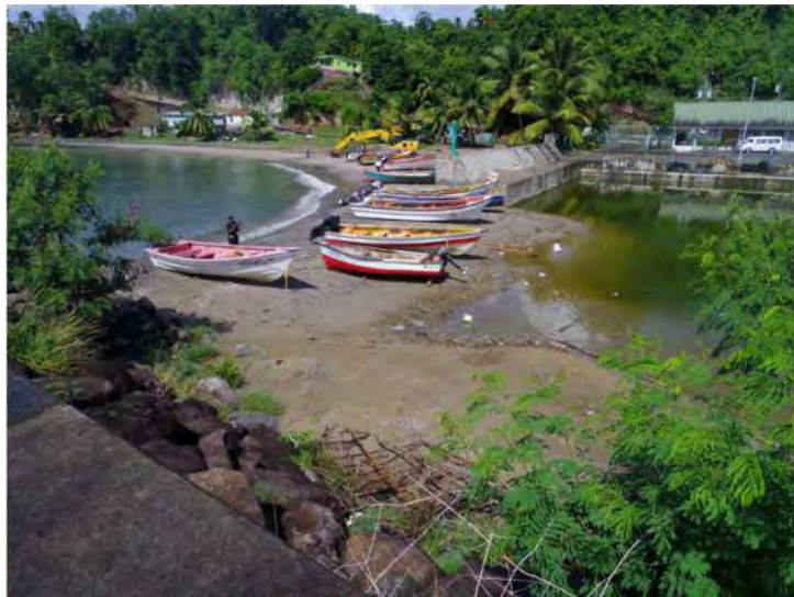
Photo 6-52 Port entrance completely blocked on November 4, 2015
