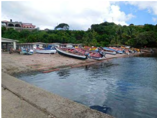
Photo 2-15 Slipway and fishing gear lockers
