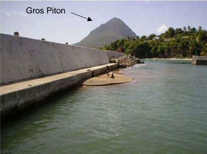
Photo 6-18 Deposition appearing on the sea surface in the fishing port taken on June 29, 2003
