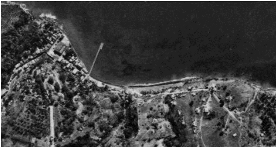
Photo 6-1 The pier in Choiseul in April 18, 1966
