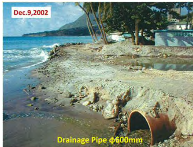
Photo 6-41 Temporary construction road and drainage
