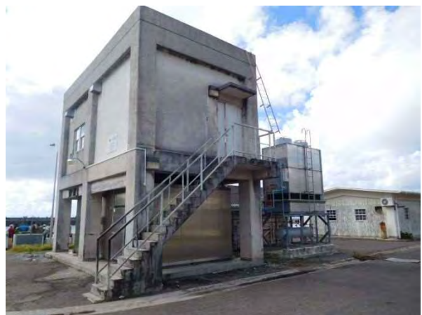
Photo 2-18 Ice machine and ice storage building
