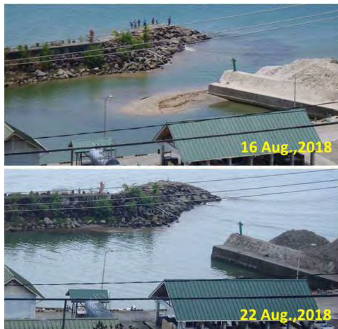
Photo 2-82 Comparison of before and after dredging work by backhoe
