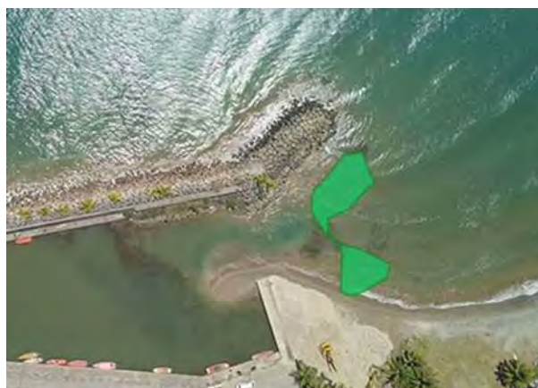
Figure 6-10 The cobble stone accumulation area in the port entrance on August 13, 2018
