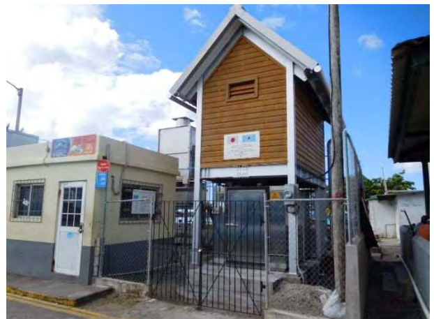
Photo 2-32 Ice machine and ice storage
