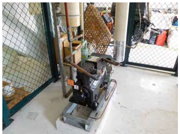
Photo 2-28 Compressor for ice machine
