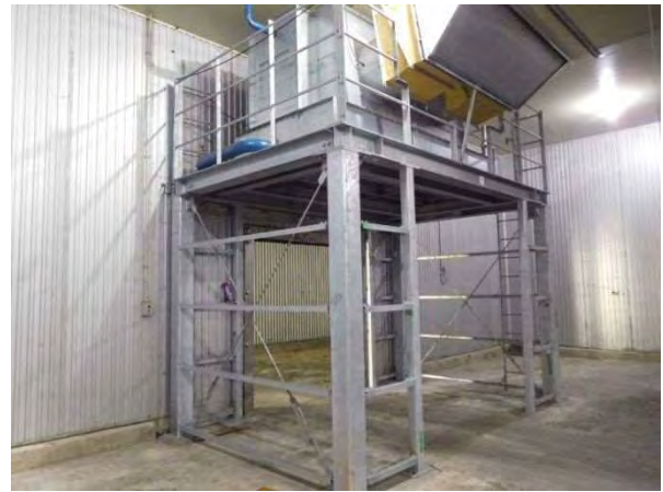
Photo 2-22 Cooling unit for cold storage
