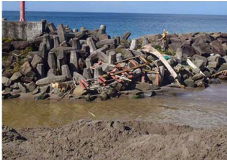
Photo 7-7 View of port entrance on November 21, 2017
