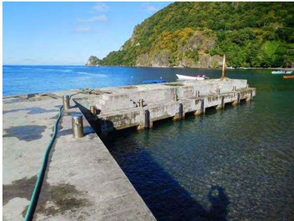
Photo 2-37 Fish landing jetty
