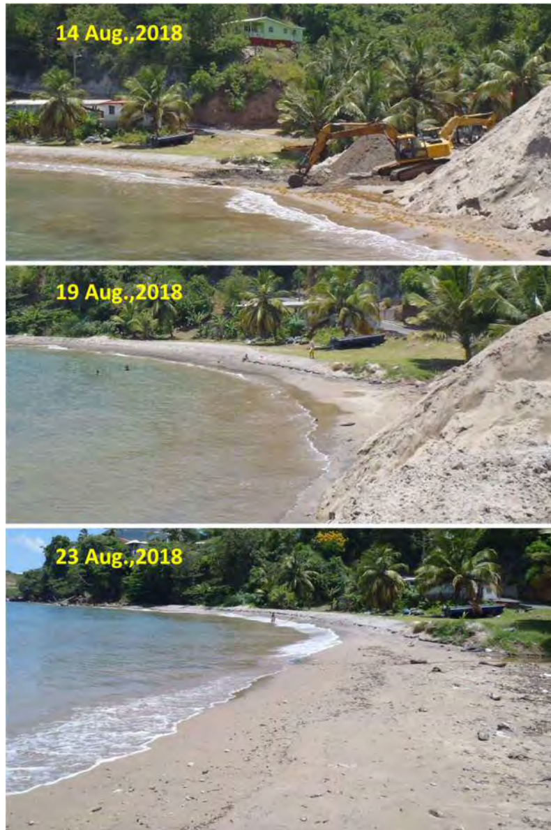
Photo 2-78 Recovery of excavation trace
