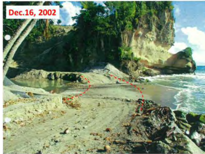
Photo 6-40 Temporary construction road at Choiseul river mouth
