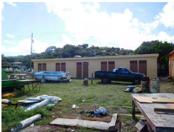
Photo 2-59 New fishing gear lockers (Constructed by the Government of Saint Lucia)
