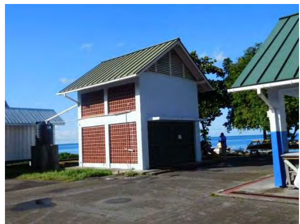
Photo 2-42 Ice machine and ice storage
