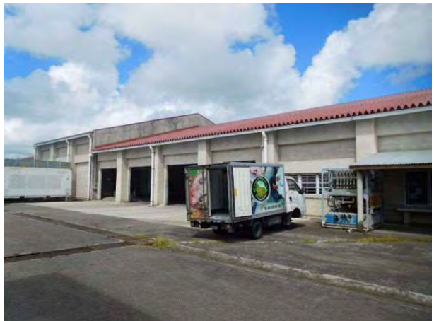
Photo 2-16 Cold storage building
