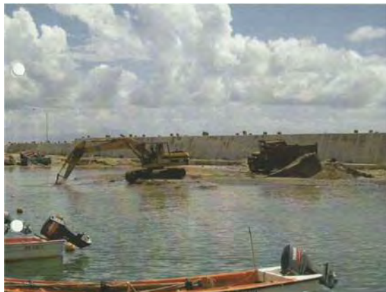
Photo 7-4 Dredging work in the port during Stage 1 on September 21, 2004
