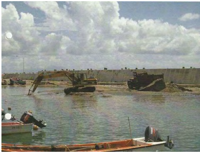
Photo 6-21 Dredging work by backhoe on September 21, 2004
