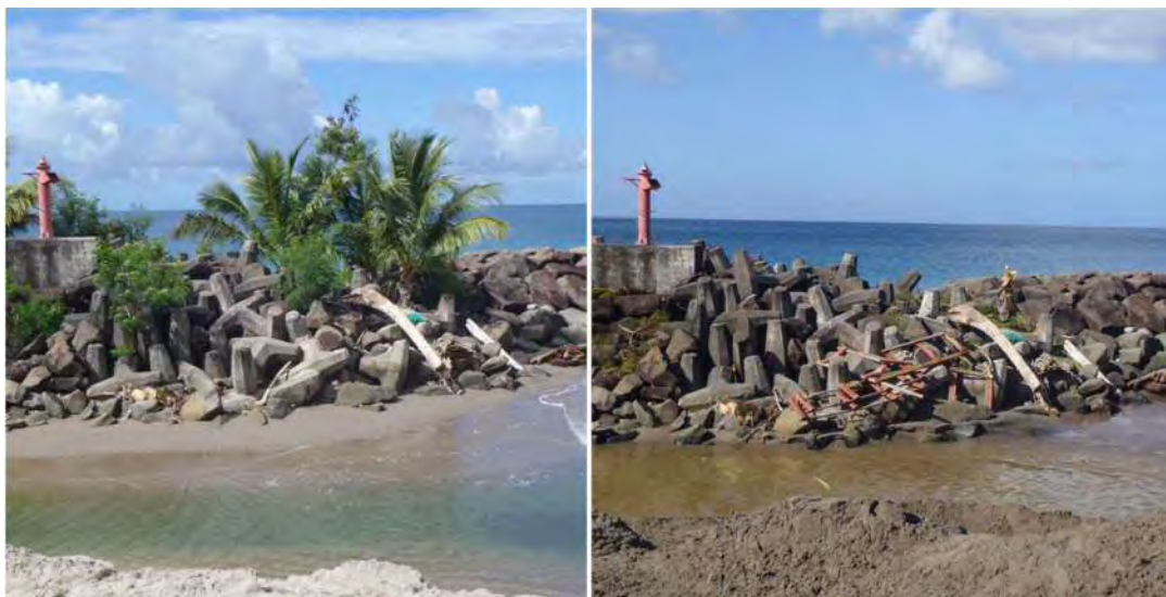
Photo 2-69 Port entrance, November 2017: Left 18th (Saturday), Right 21st (Tuesday)
