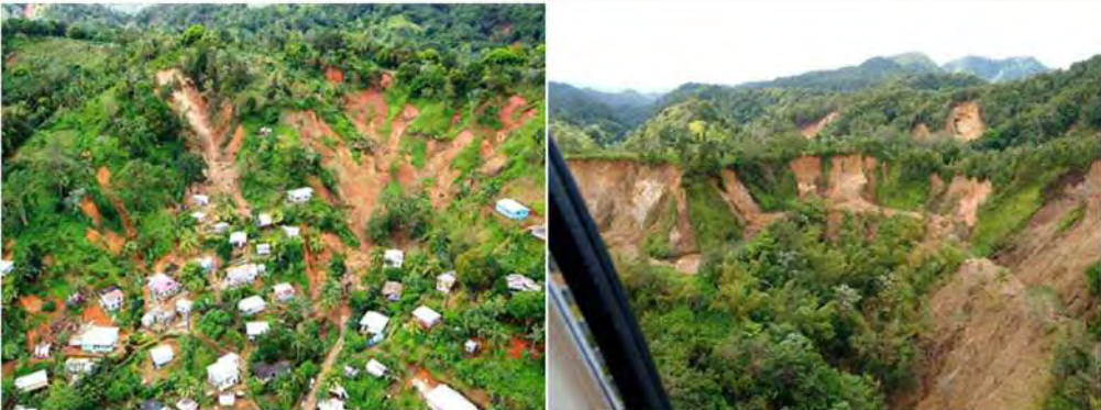
Photo 6-56 Massive hillside collapse due to hurricane Tomas
