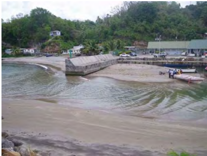
Photo 6-48 The port entrance (May 9, 2009)
