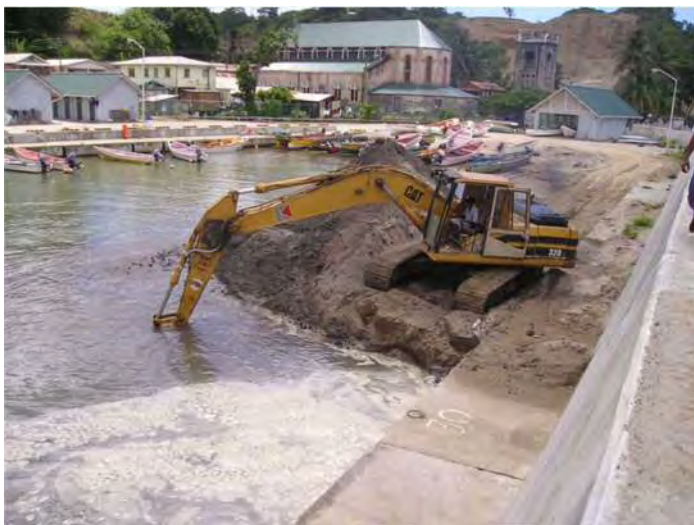
Photo 6-22 Dredging work by backhoe on October 19, 2004
