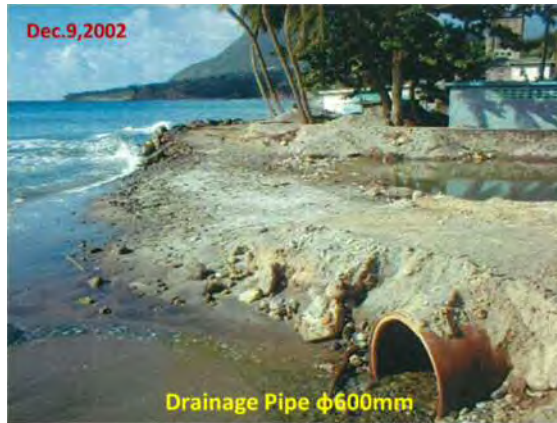
Photo 6-27 Temporary road and drainage pipe in the Choiseul river mouth
