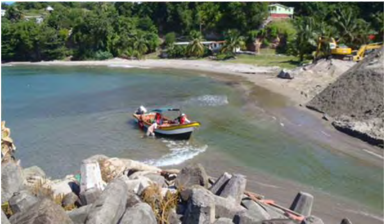
Photo 2-71 The remaining shallow area after dredging by backhoe on November 24, 2017
