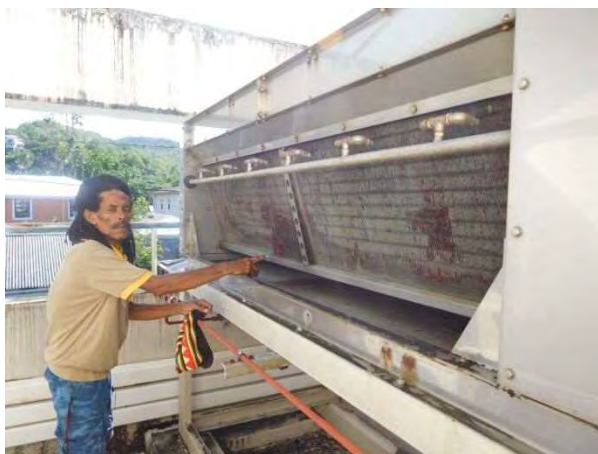
Photo 2-29 Broken condenser
