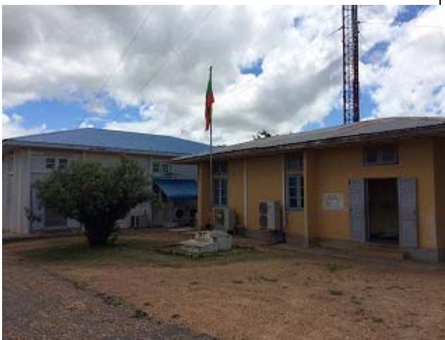
Thabeikkyin Transmitting Station
