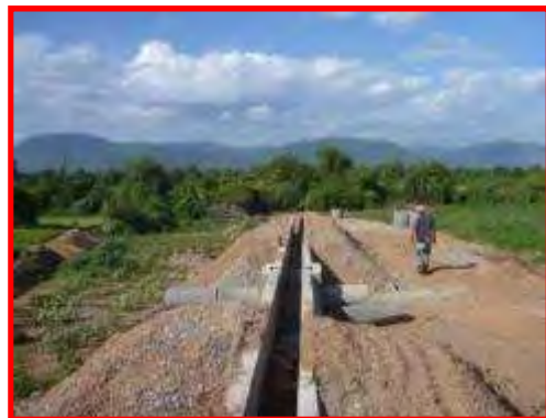
③ Nearly completed
