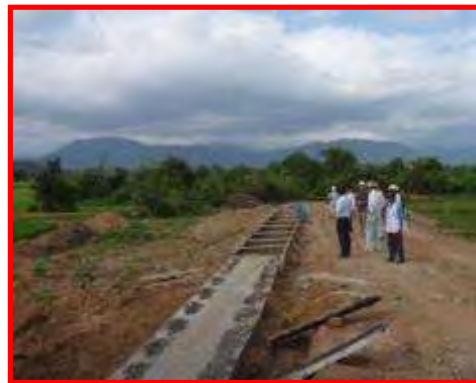
② Under construction
