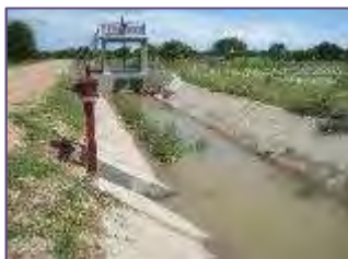
Primary canal D8
