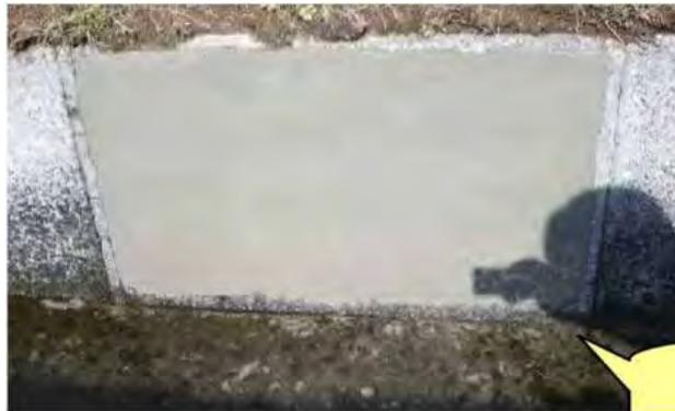
• Protected 3 days after construction and do not pass water
