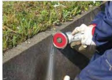
Cut the width of about 1 cm and the depth of about 2 cm along the crack
