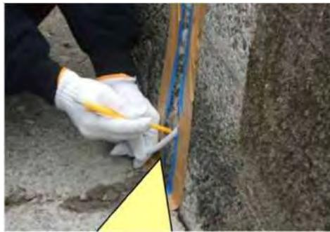
• Install the backup material at a depth of about half of the joint width
